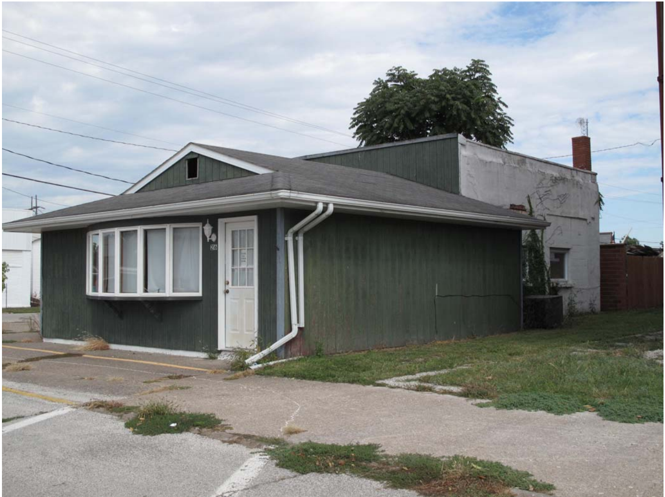
Photograph 92-00507-002 - West and south elevations, looking northeast (McCarley, September 20, 2011)
