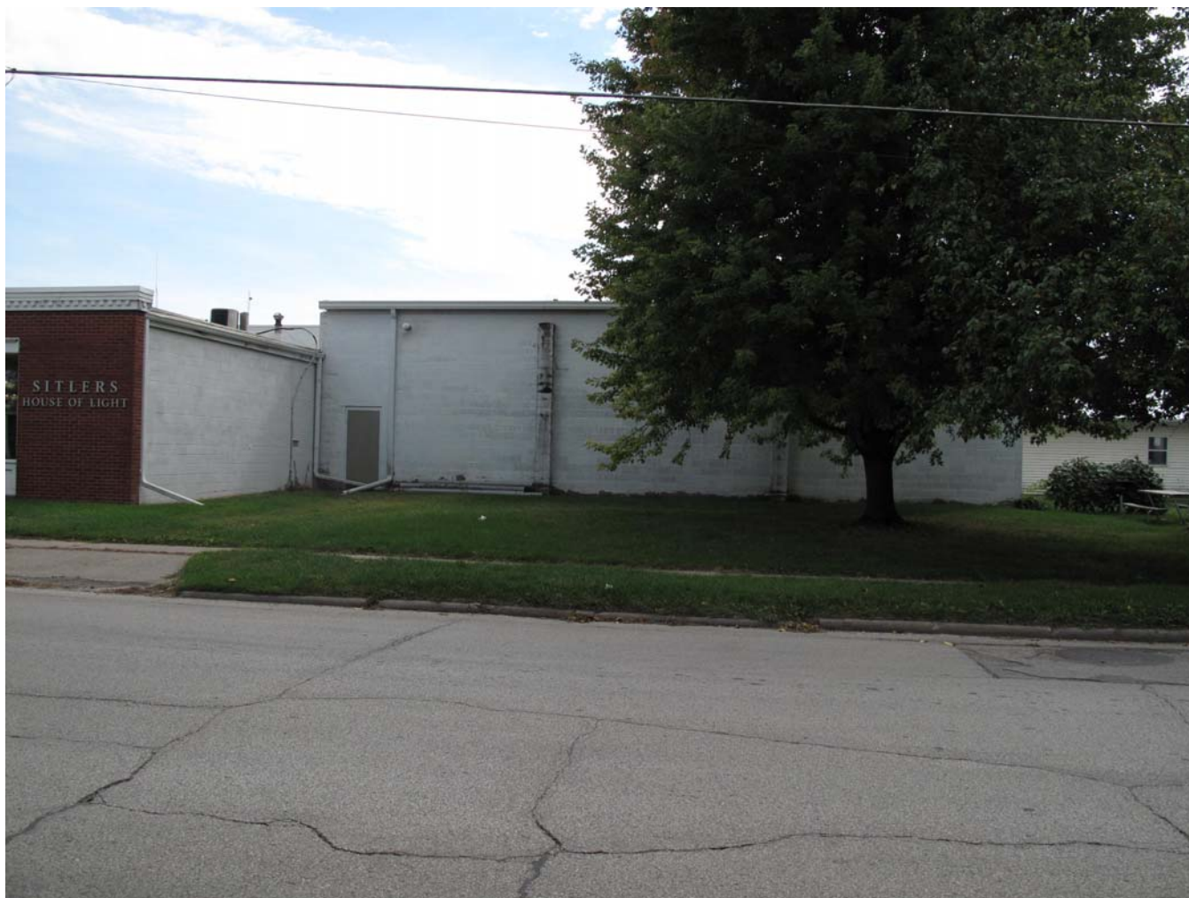
Photograph 92-00591-001 - North elevation, looking south (McCarley, September 20, 2011)
