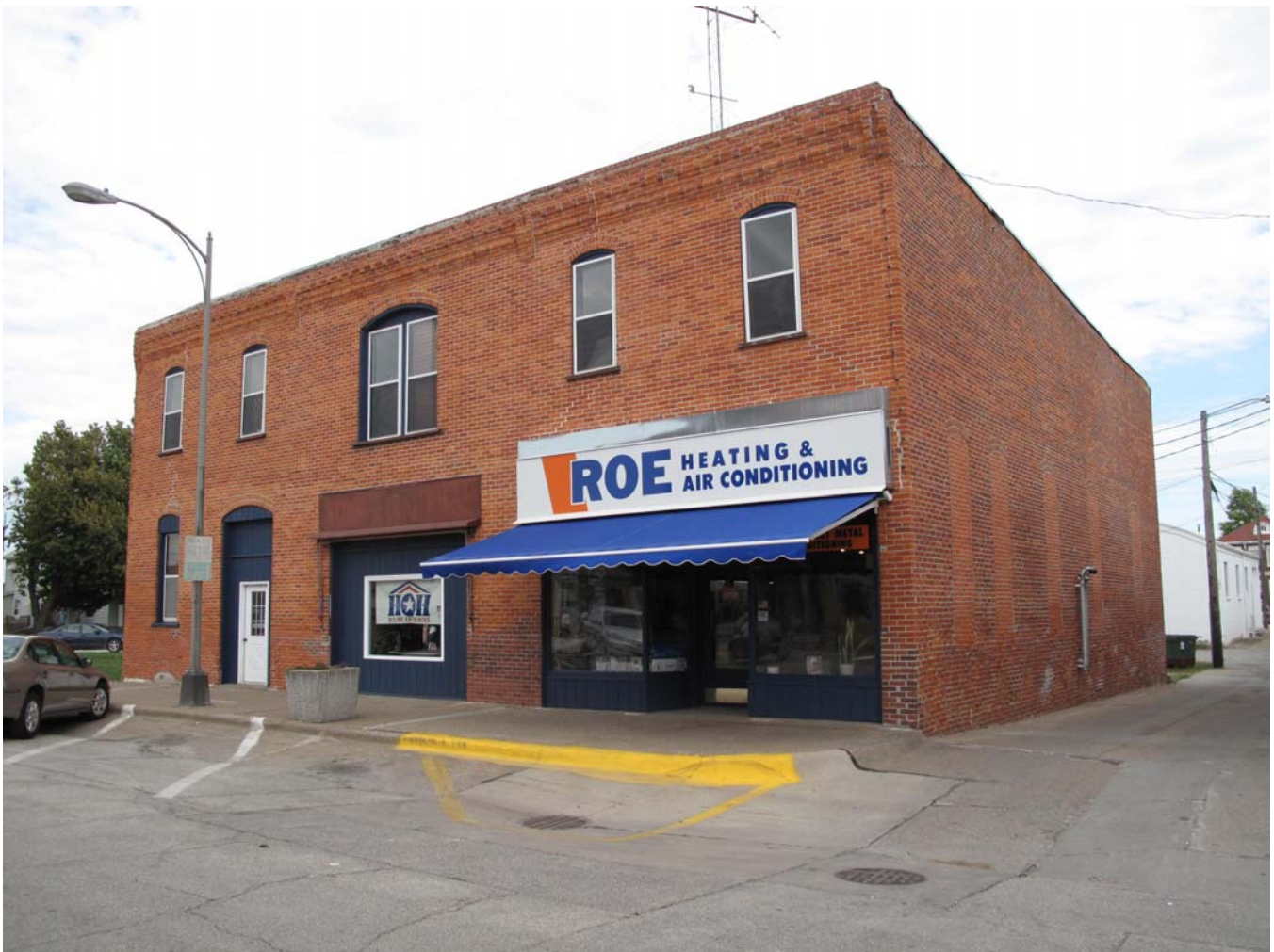
Photograph 92-00501-001 - West and south elevations, looking northeast (McCarley, September 20, 2011)
