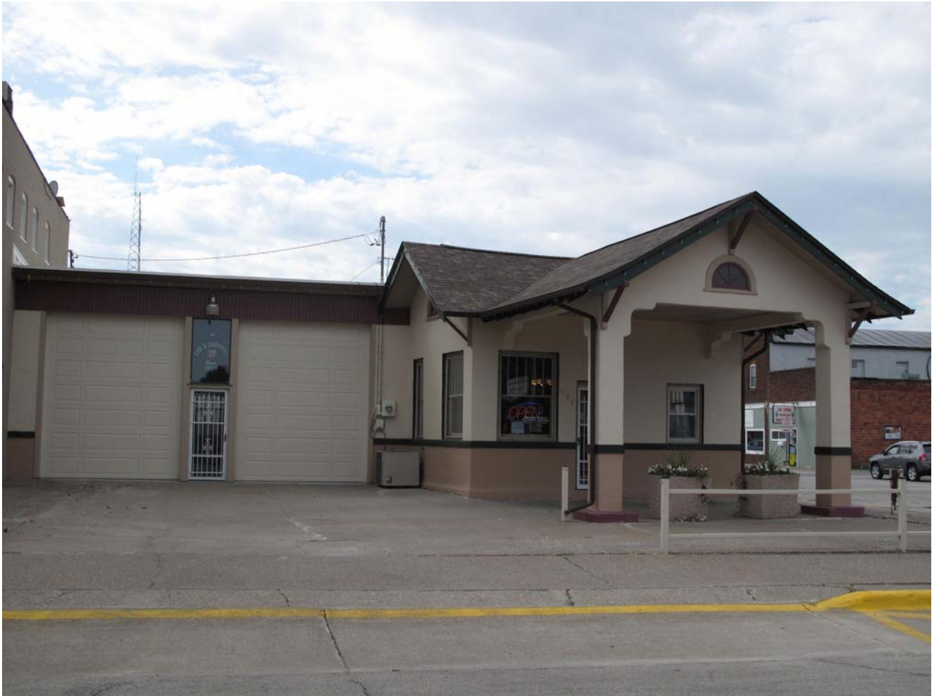
Photograph 92-00504-003 - East elevation, looking west (McCarley, September 20, 2011)
