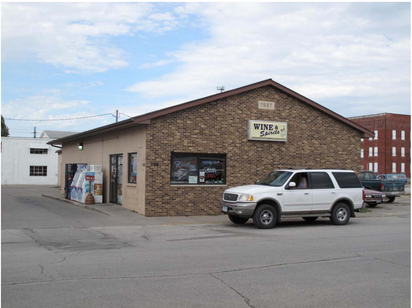
Photograph 92-00580-001 - West and south elevations, looking northeast (McCarley, September 20, 2011)
