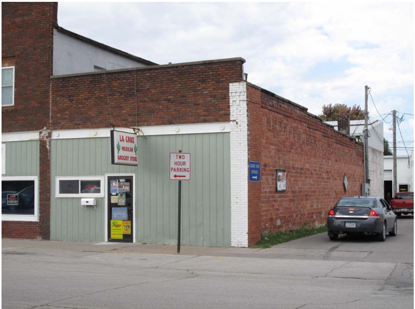
Photograph 92-00583-001 - South and east elevations, looking northwest (McCarley, September 20, 2011)
