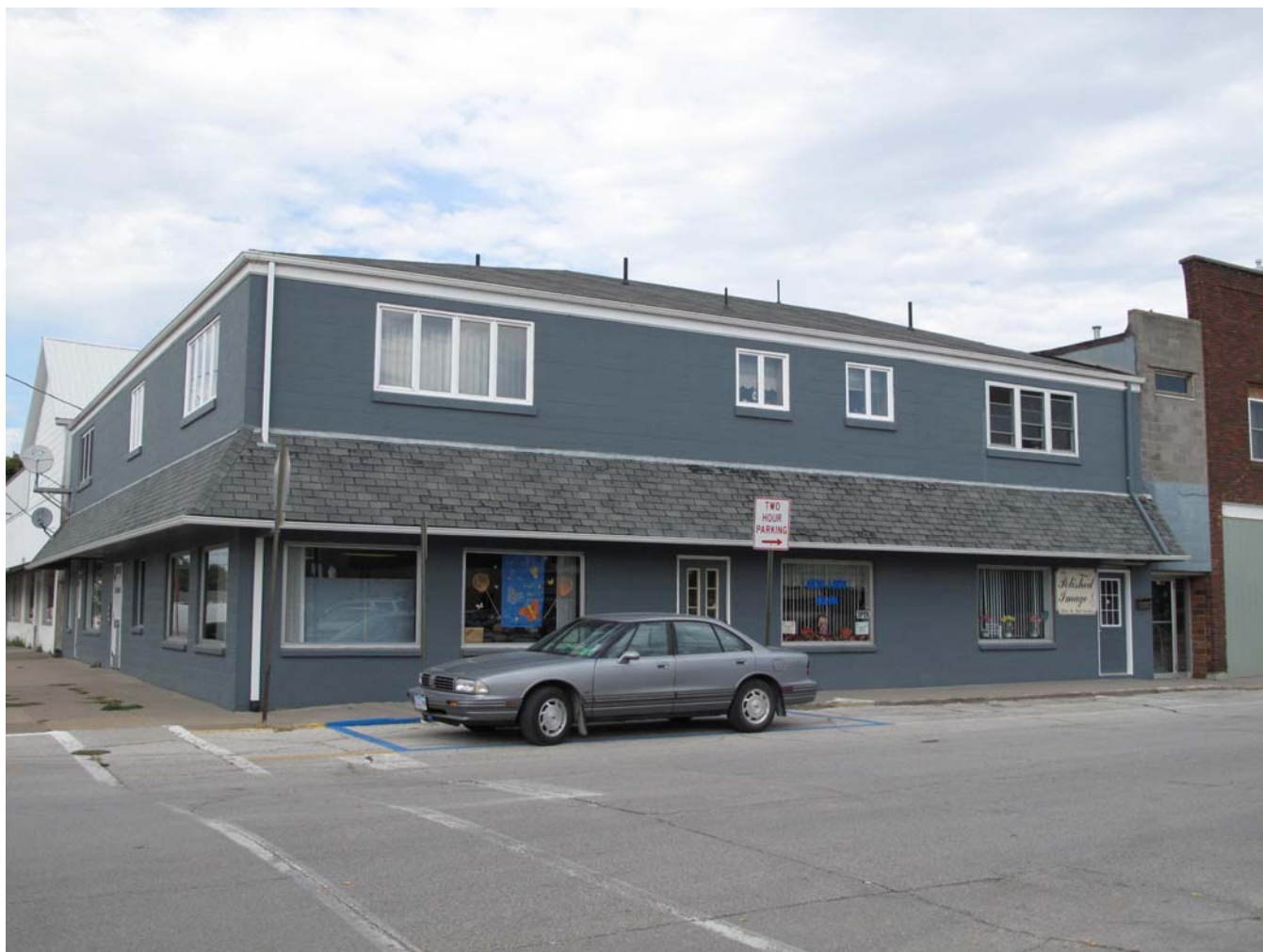
Photograph 92-00586-001 - West and south elevations, looking northeast (McCarley, September 20, 2011)
