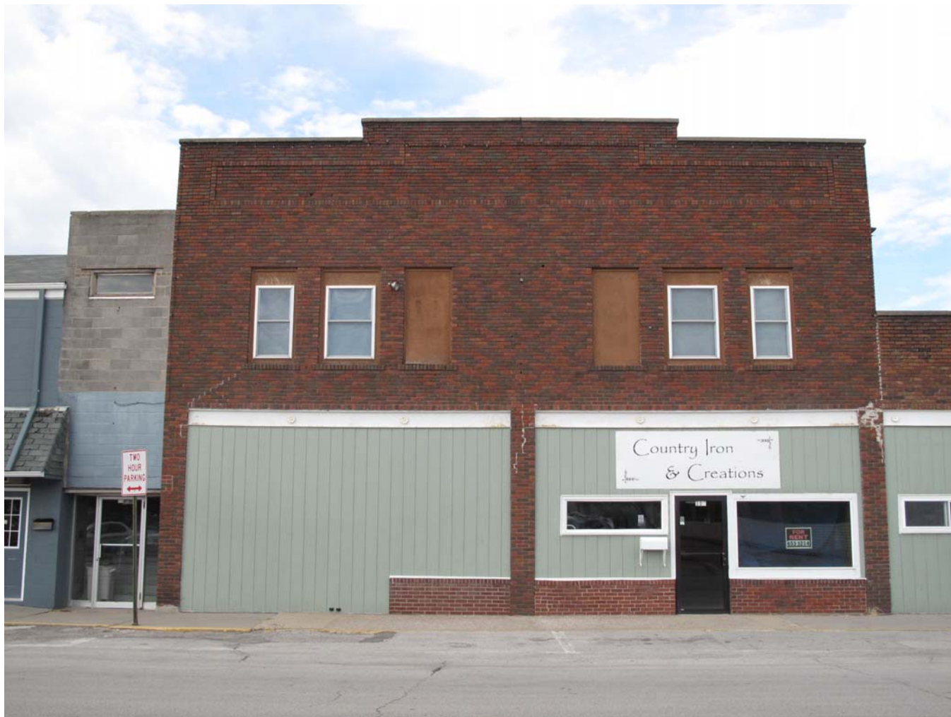
Photograph 92-00582-002 - South facade, looking north (McCarley, September 20, 2011)
