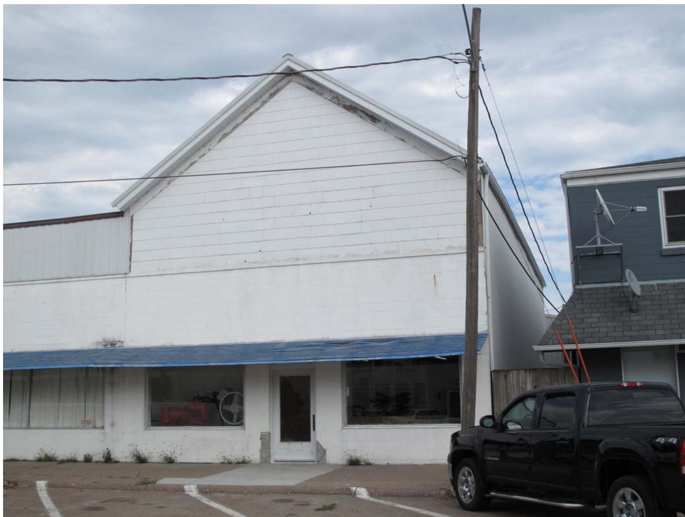
Photograph 92-00553-001 - West and south elevations, looking east-northeast (McCarley, September 20, 2011)
