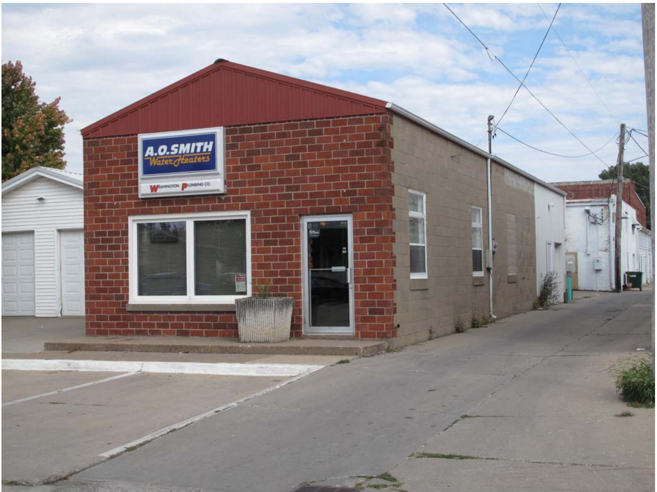
Photograph 92-00556-001 - West and south elevations, looking northeast (McCarley, September 20, 2011)
