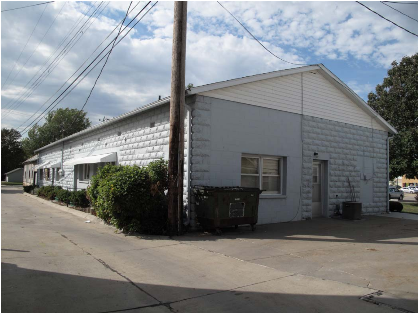
Photograph 92-00592-003 - South and east elevations of original section, looking northwest (McCarley, September 20, 2011)
