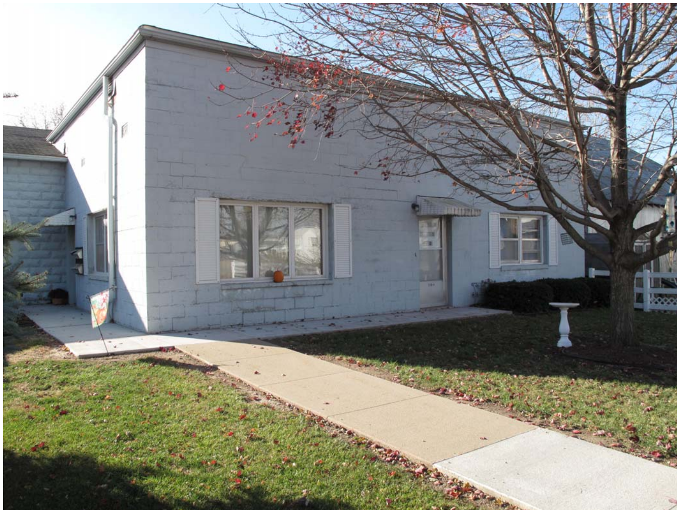
Photograph 92-00592-002 - North elevation of west addition, looking southwest (McCarley, November 15, 2011)
