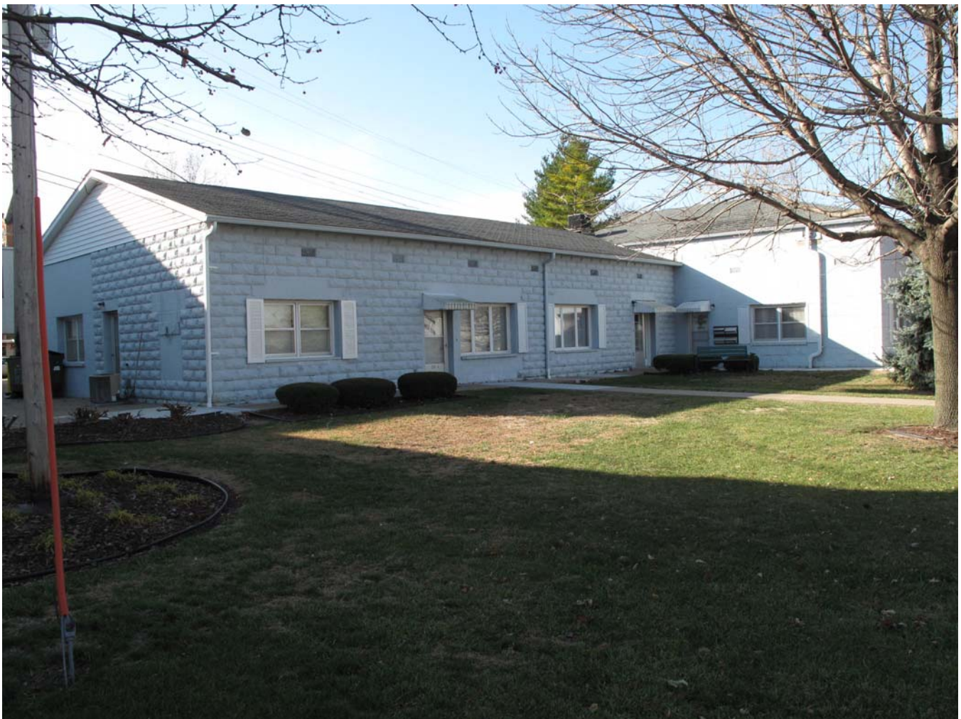
Photograph 92-00592-001 - East and north elevations of original section, looking southwest (McCarley, November 15, 2011)
