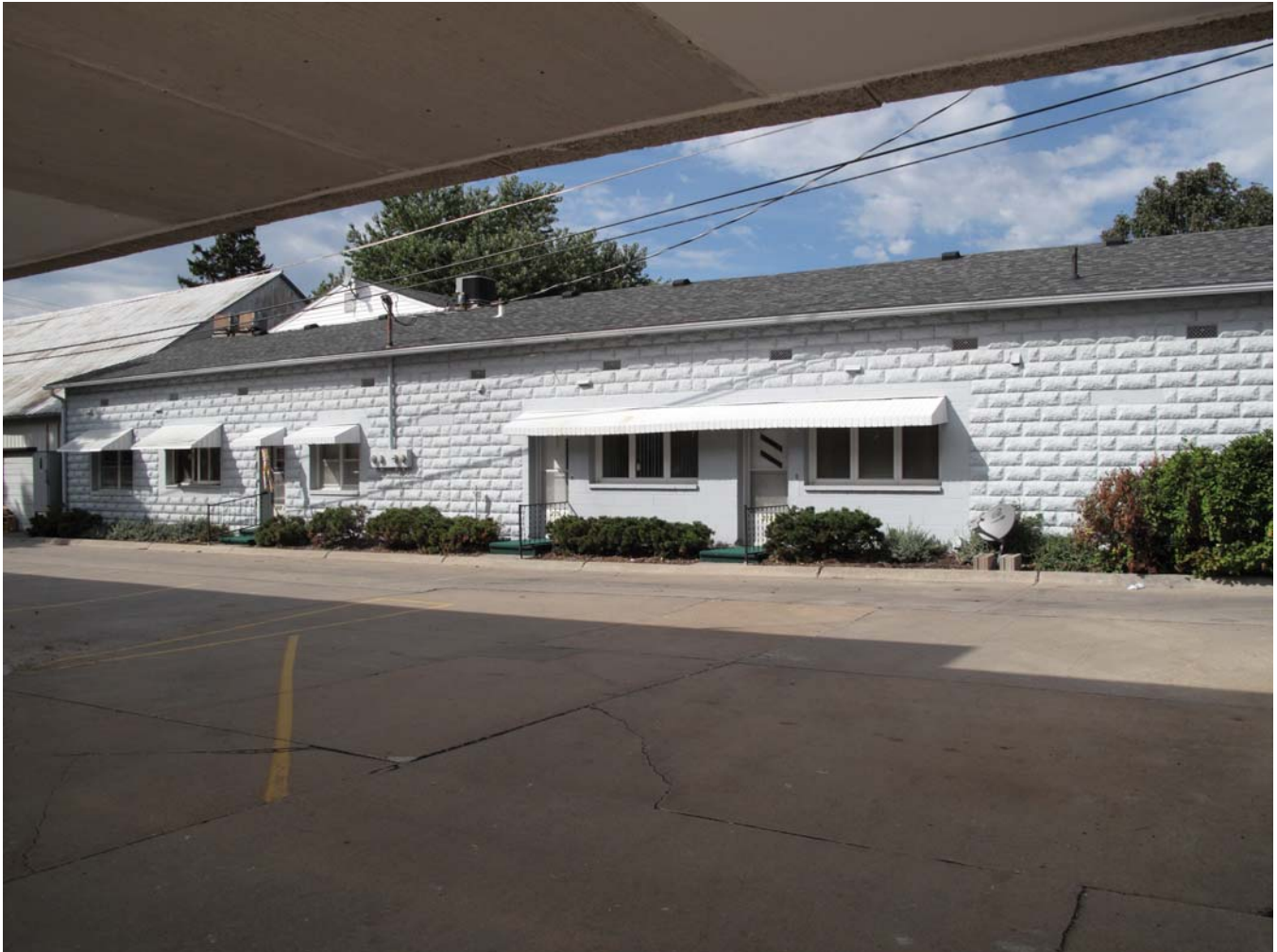
Photograph 92-00592-004 - South elevation of original section, looking north (McCarley, September 20, 2011)
