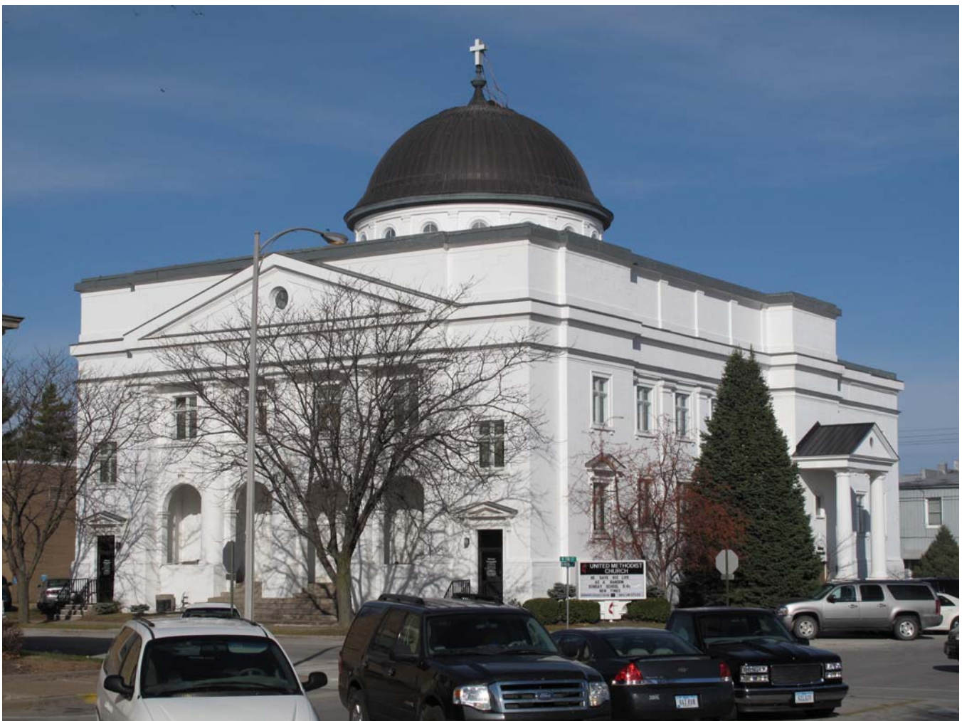
Photograph 92-00346-001 - South and east elevations, looking northwest (McCarley, November 15, 2011)
