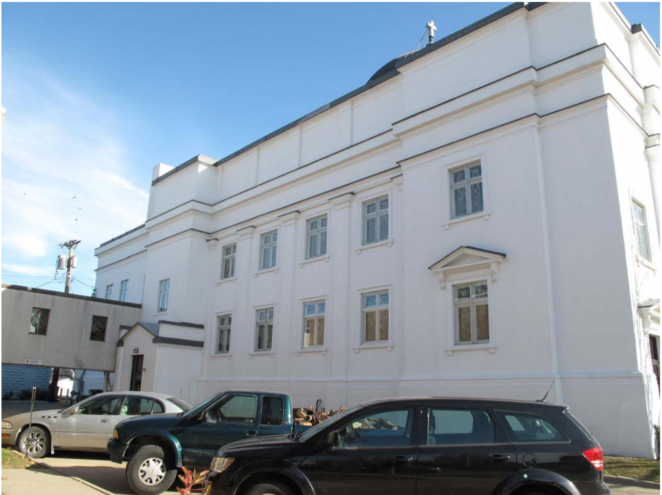
Photograph 92-00346-005 - West elevation, looking northeast (McCarley, November 15, 2011)
