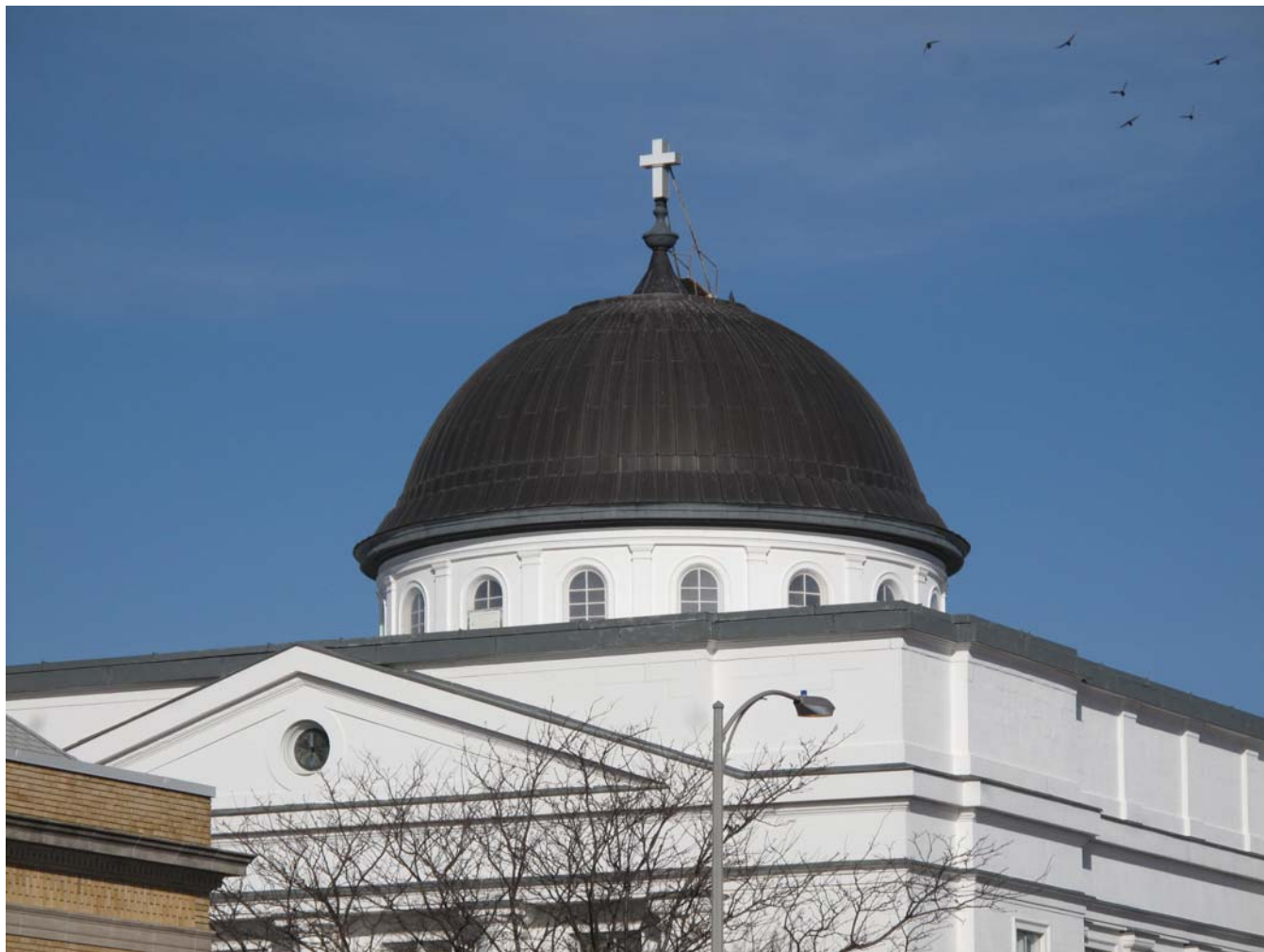
Photograph 92-00346-003 - Detail of dome, looking northwest (McCarley, November 15, 2011).
