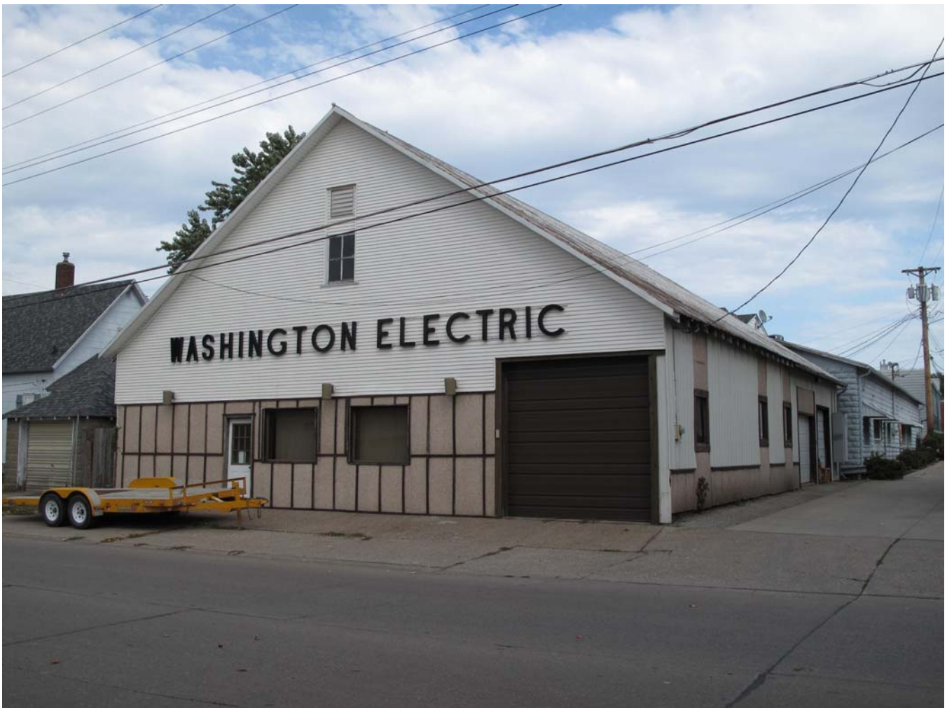
Photograph 92-00495-001 - West and south elevations, looking northeast (McCarley, September 20, 2011)
