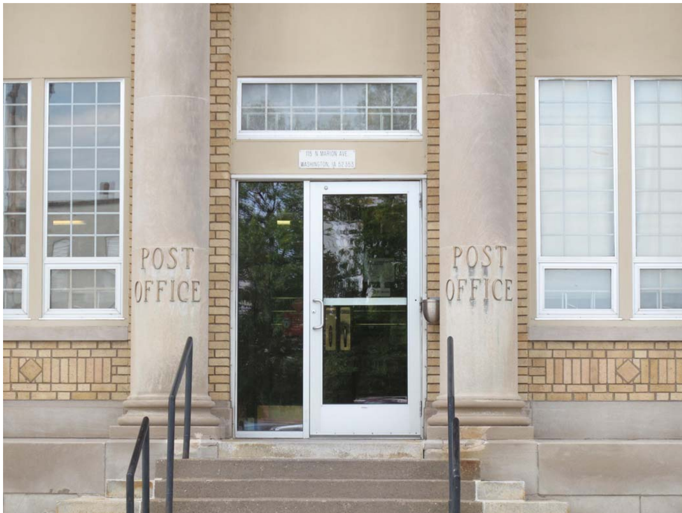
Photograph 92-00165-004 - Detail of east elevation, looking west (McCarley, September 20, 2011)
