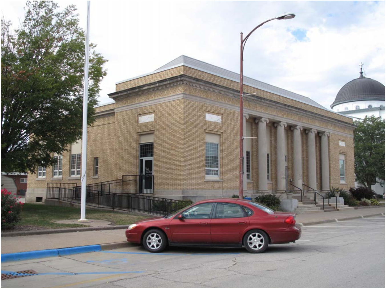
Photograph 92-00165-002 - South and east elevations, looking northwest (McCarley, September 20, 2011)
