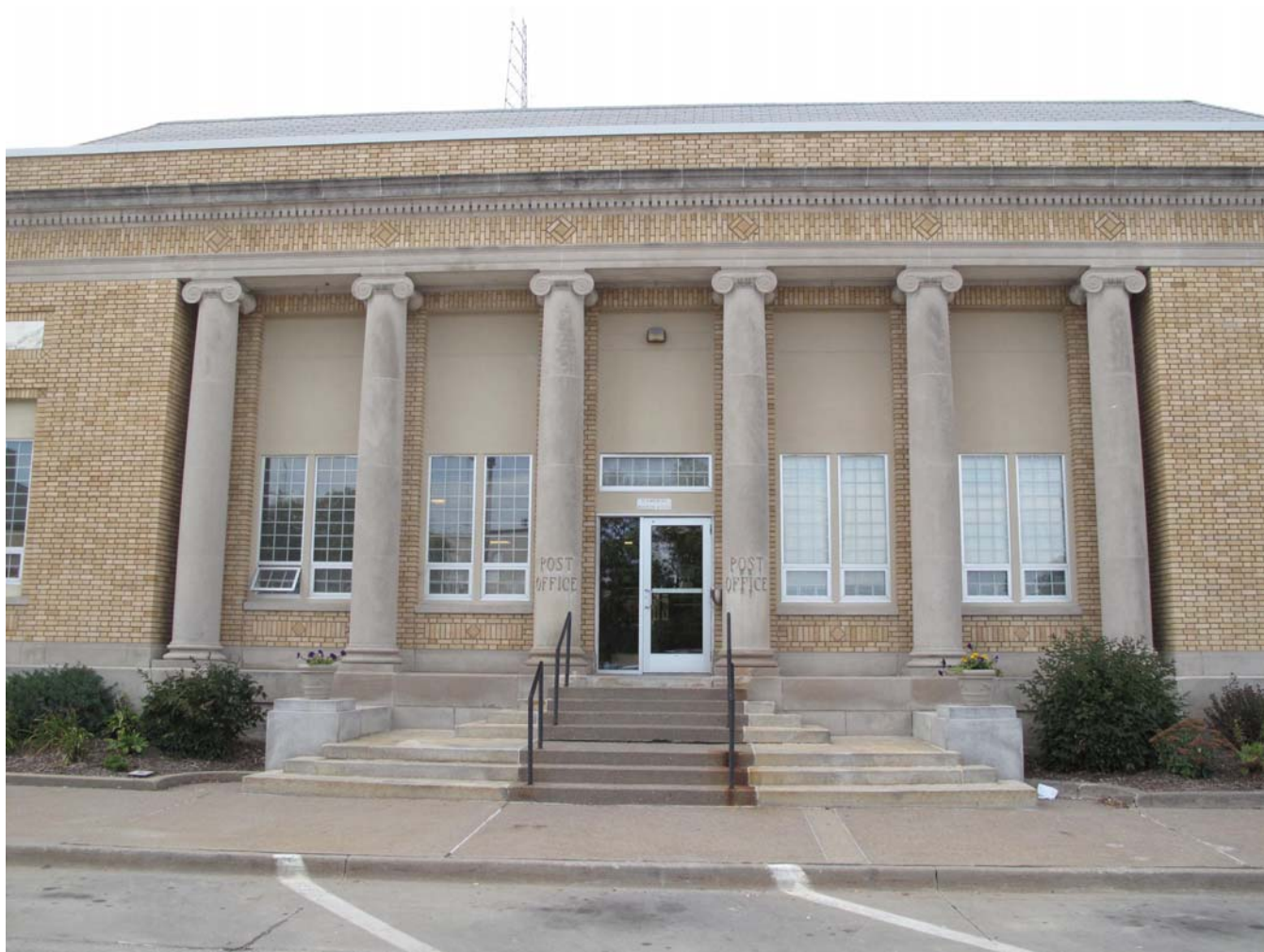
Photograph 92-00165-003 - East elevation, looking west (McCarley, September 20, 2011)
