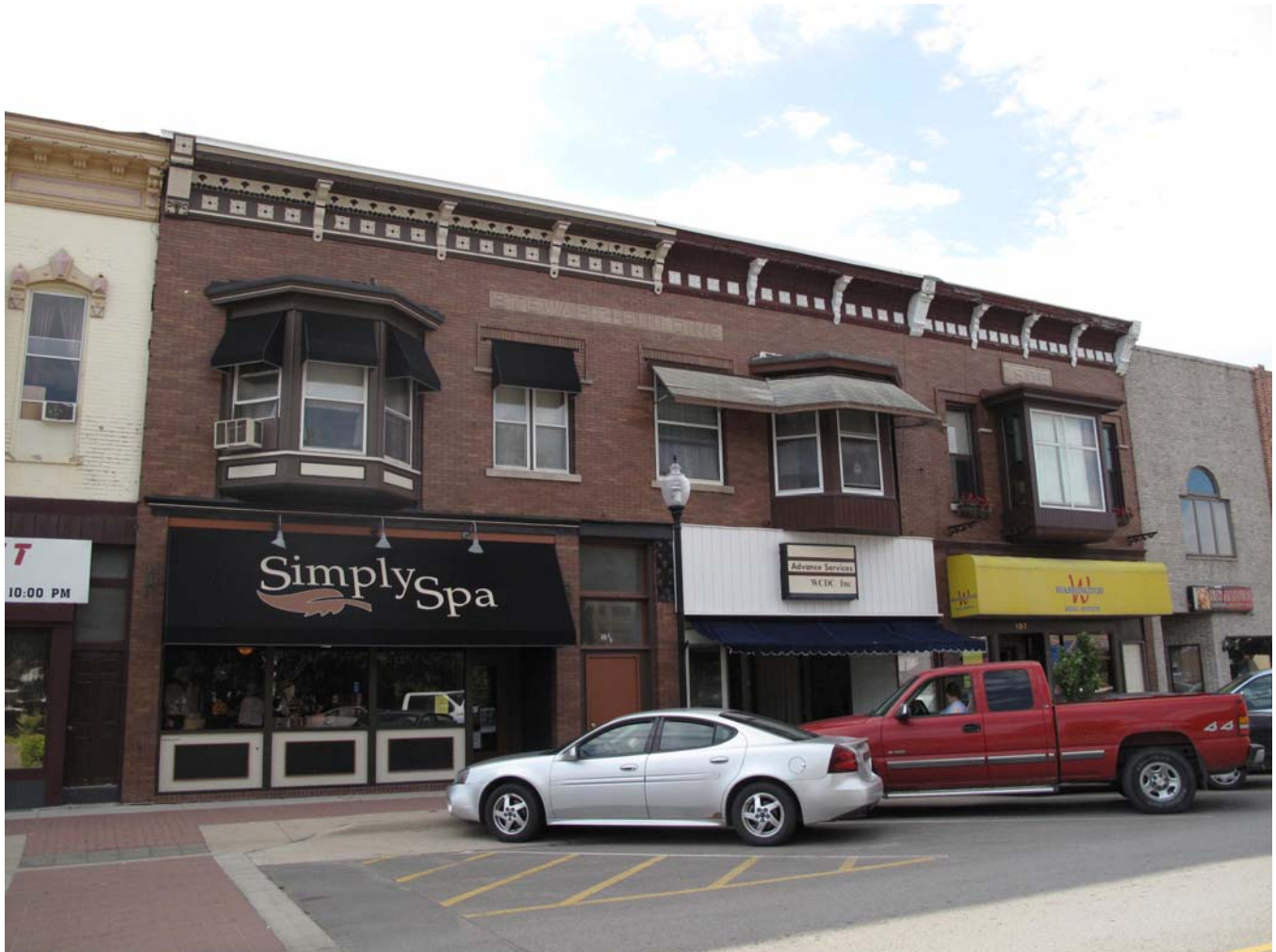
Photograph 92-00561-002 - East elevation of Stewart Building (111-109) and Mount Building (107), looking northwest (McCarley, September 20, 2011)
