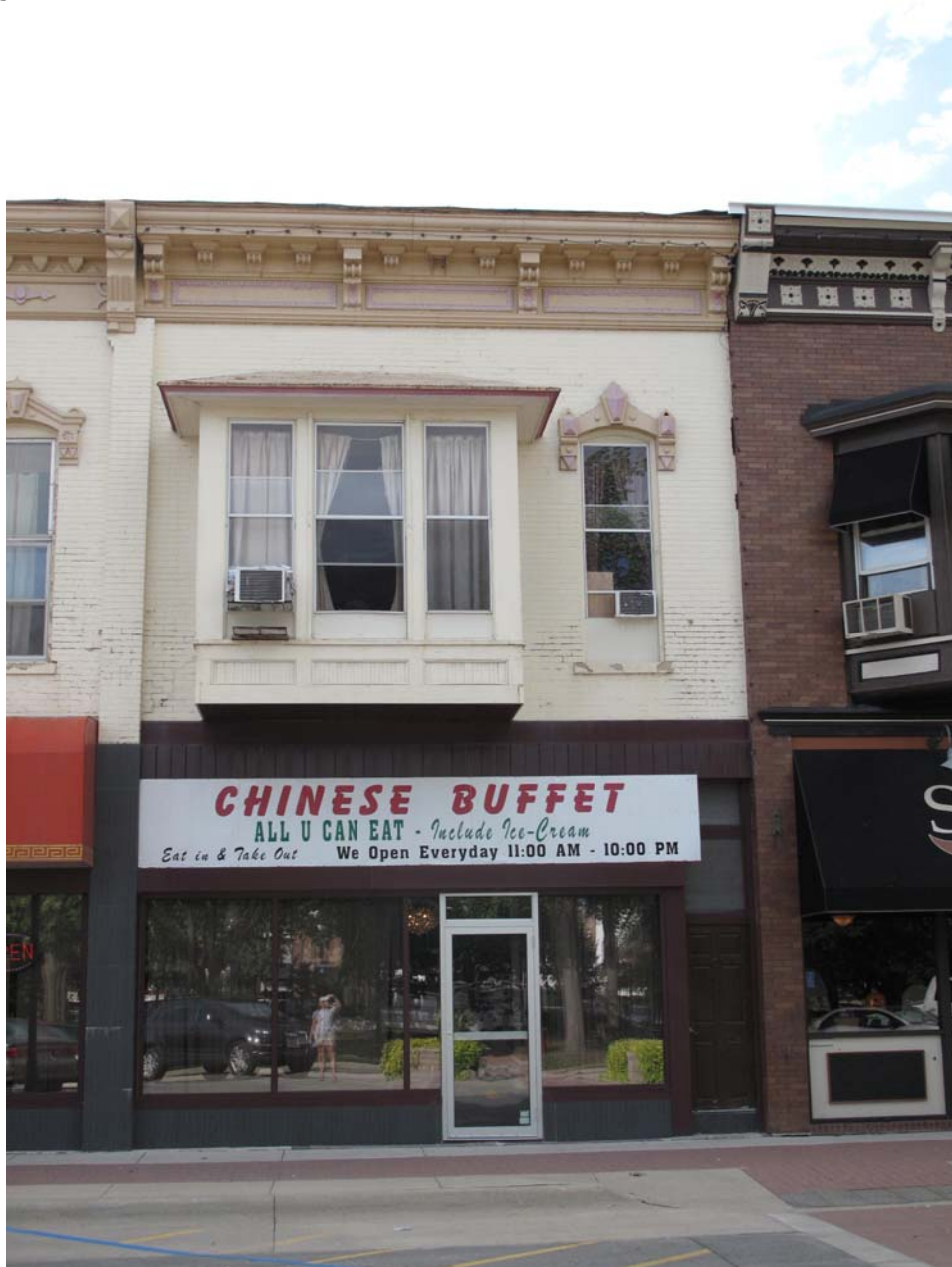
Photograph 92-00562-001 - East elevation, looking west (McCarley, September 2011)
