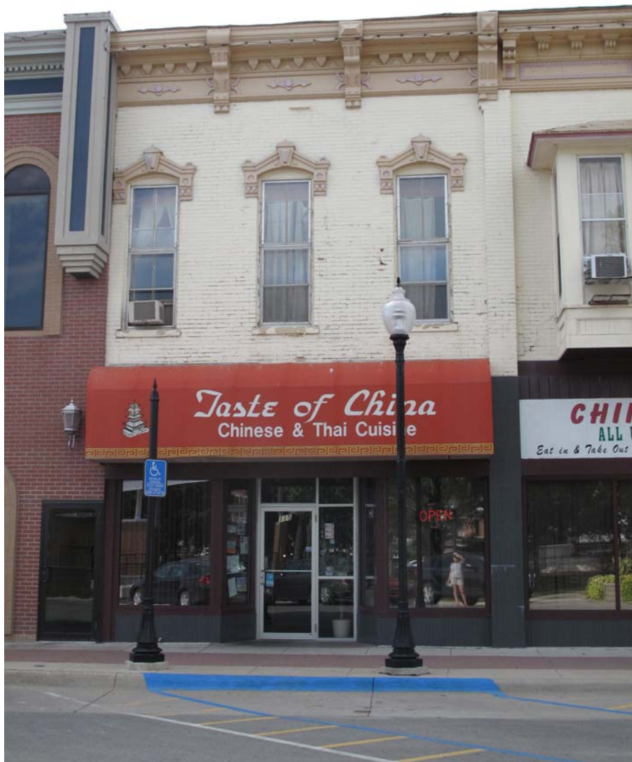
Photograph 92-00563-001 - East elevation, looking west (McCarley, September 20, 2011)
