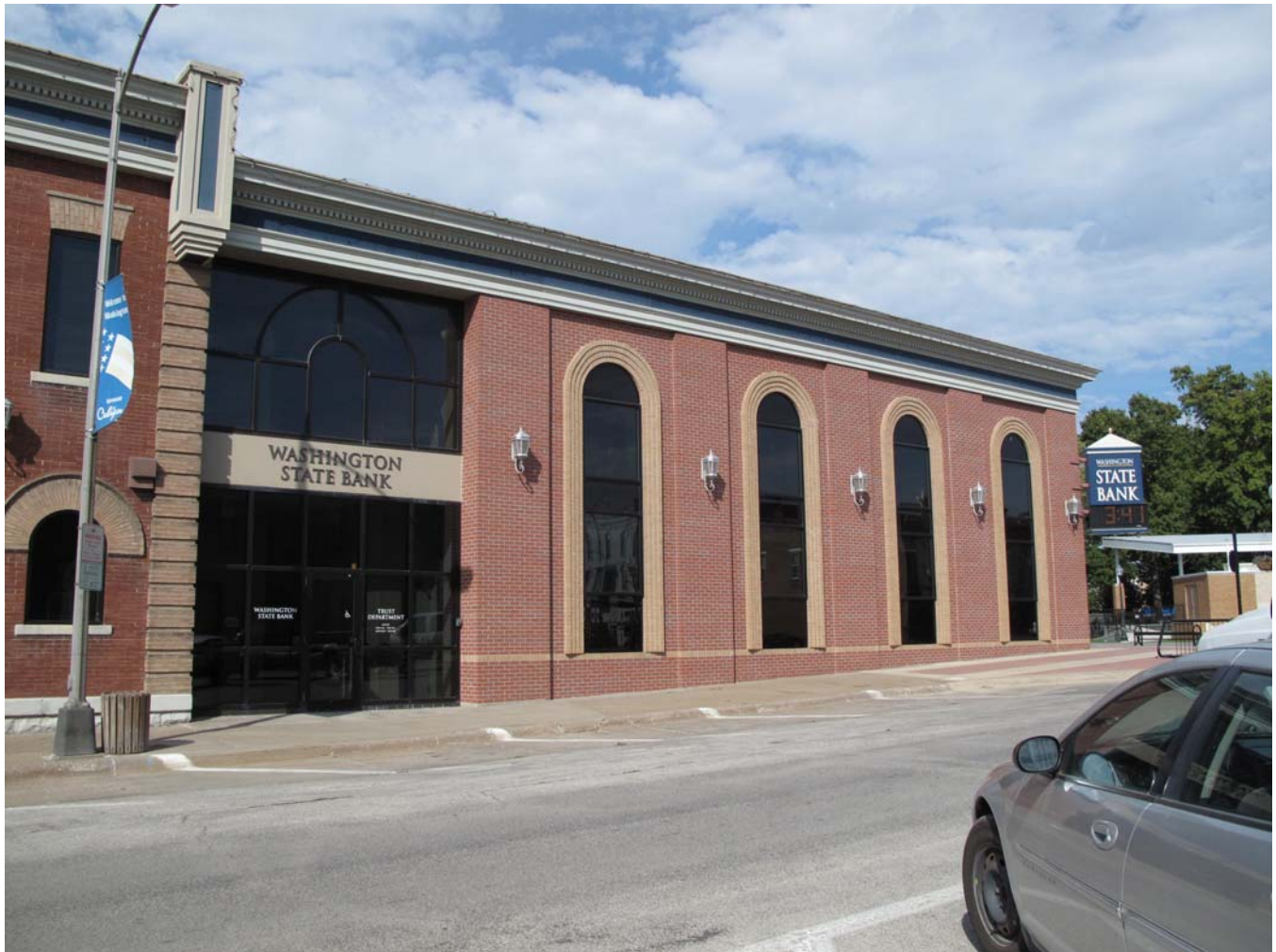
Photograph 92-00565-002 - South elevation, looking northeast (McCarley, September 20, 2011)
