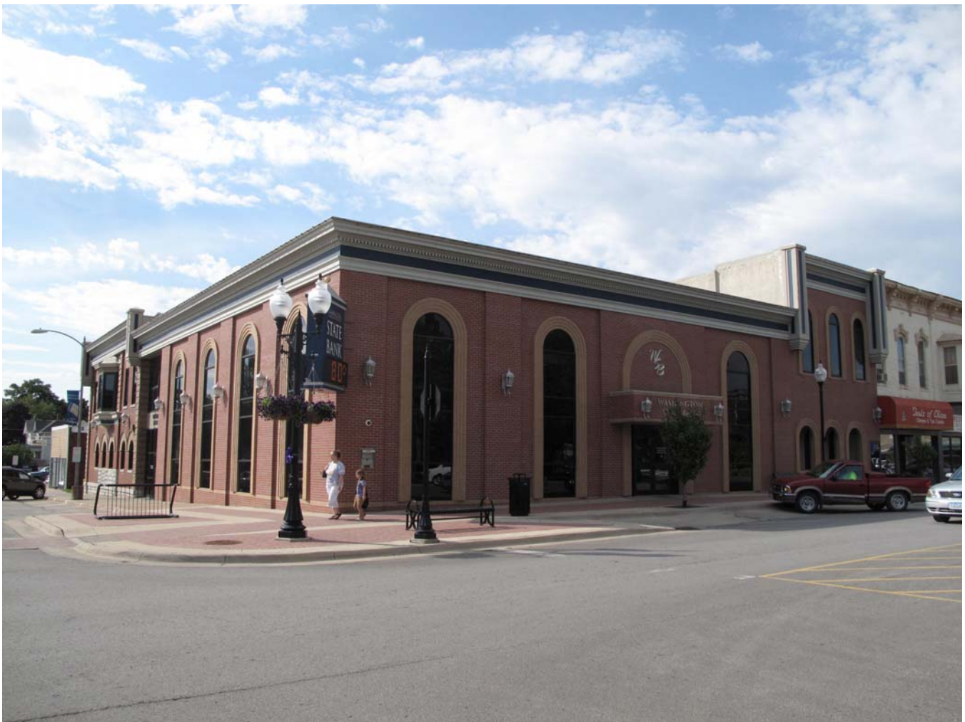
Photograph 92-00565-001 - South and east elevations, looking northwest (McCarley, September 20, 2011)
