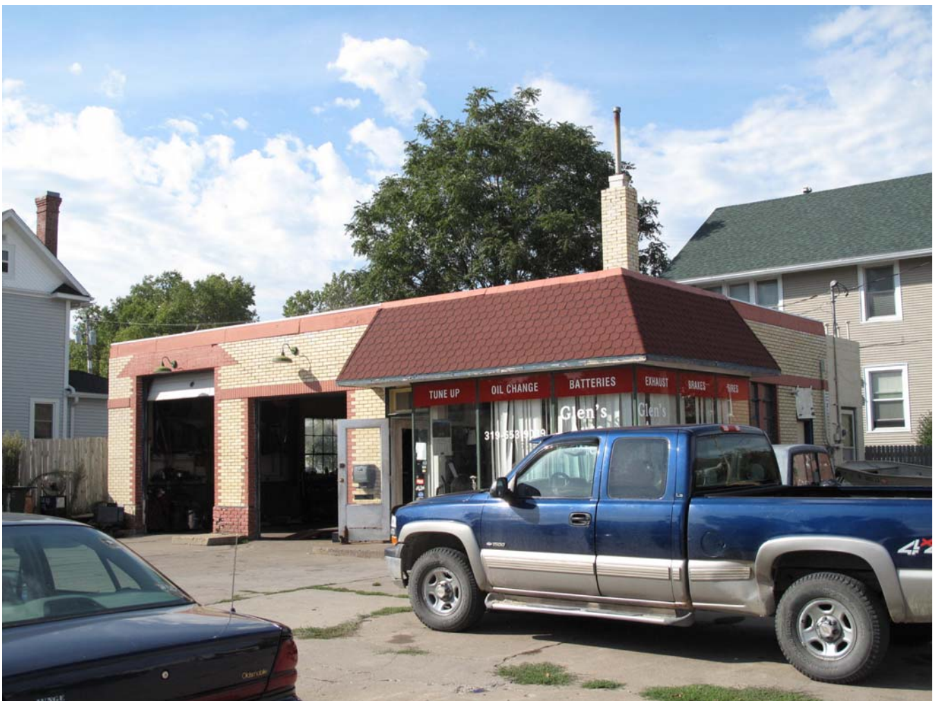
Photograph 92-00498-001 - South and east elevations, looking northwest (McCarley, September 20, 2011)
