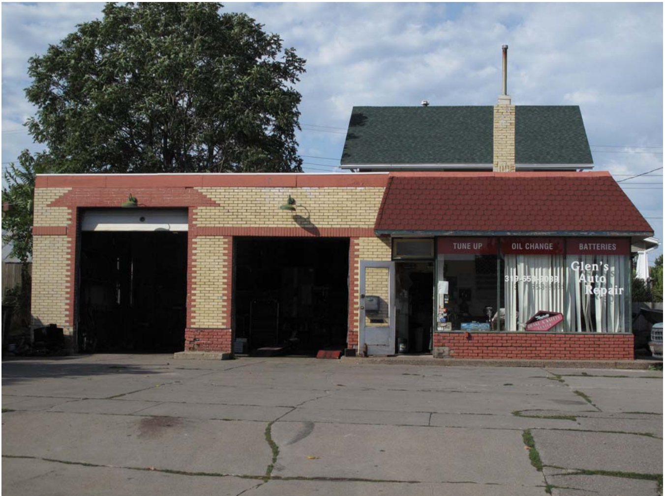
Photograph 92-00498-002 - South elevation, looking north (McCarley, September 20, 2011)
