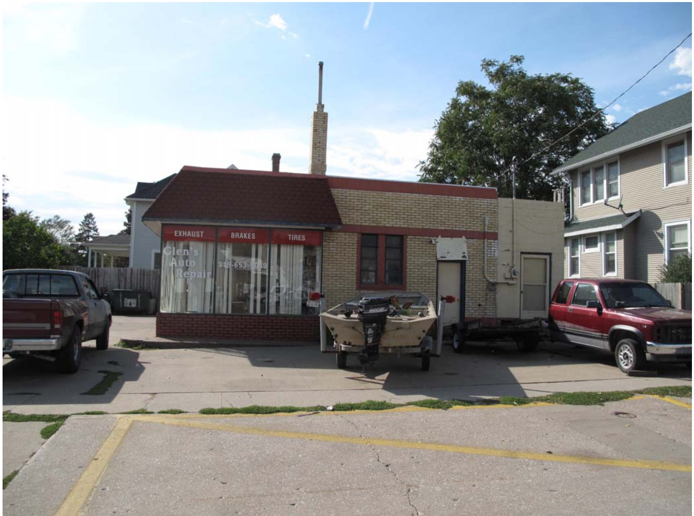
Photograph 92-00498-003 - East elevation, looking west (McCarley, September 20, 2011)
