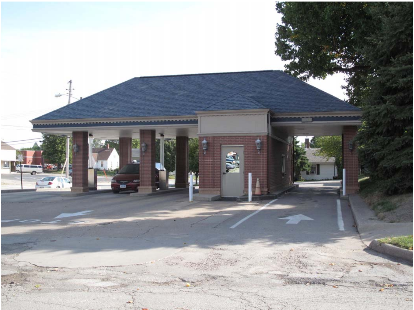
Photograph 92-00615-001 - North elevation, looking southeast (McCarley, September 20, 2011)
