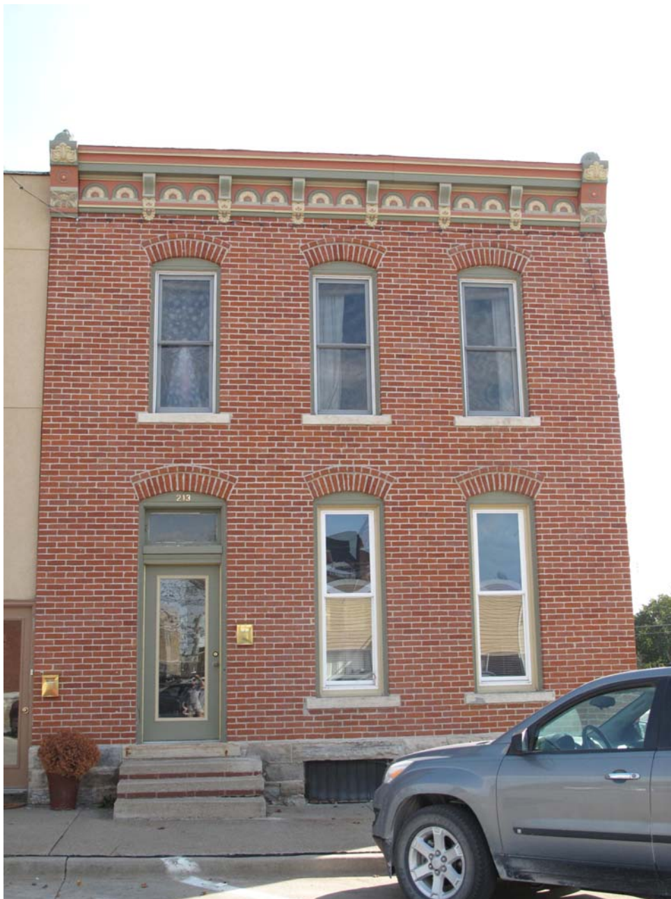
Photograph 92-00611-001 - North elevation, looking south (McCarley, September 20, 2011)
