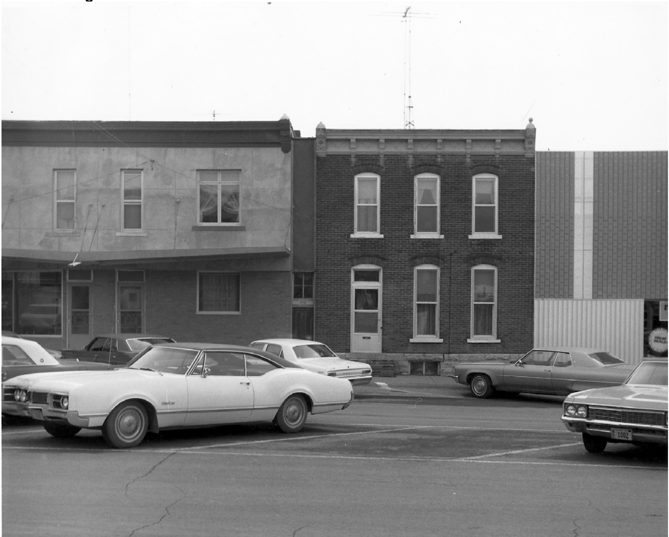
Building in 1971 (Wagner 1971)
