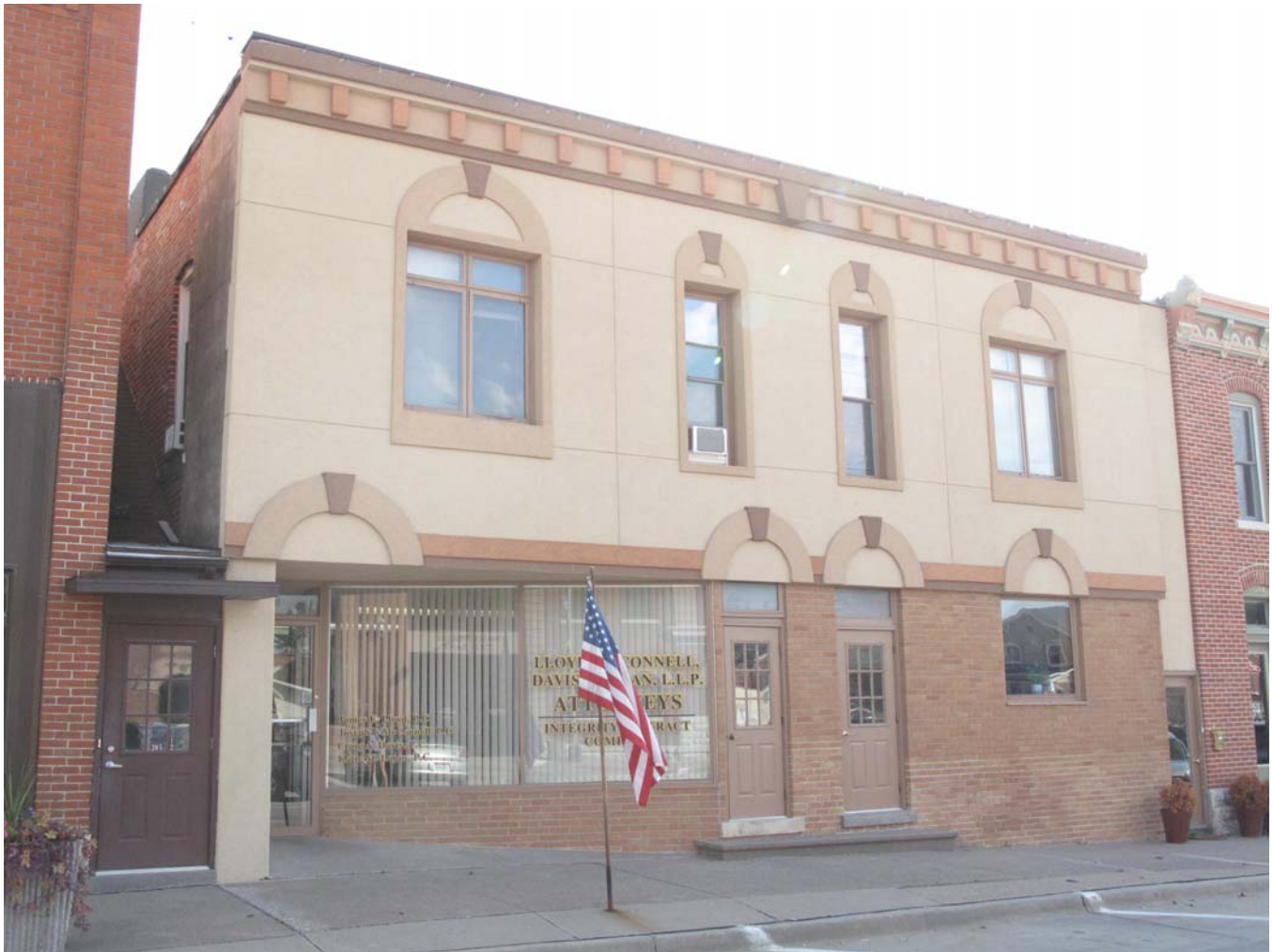
Photograph 92-00609-002 - North elevation, looking southwest (McCarley, September 20, 2011)
