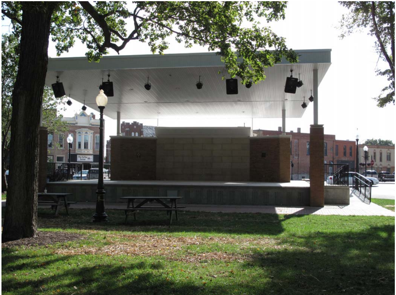
Photograph 92-00490-002 - Bandstand, looking southwest (McCarley, September 20, 2011)
