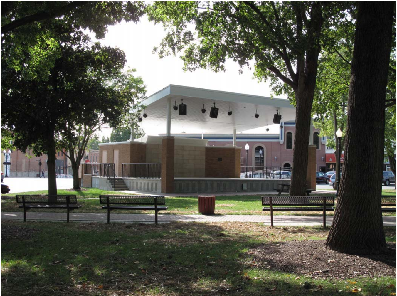
Photograph 92-00490-001 - Bandstand, looking southwest (McCarley, September 20, 2011)
