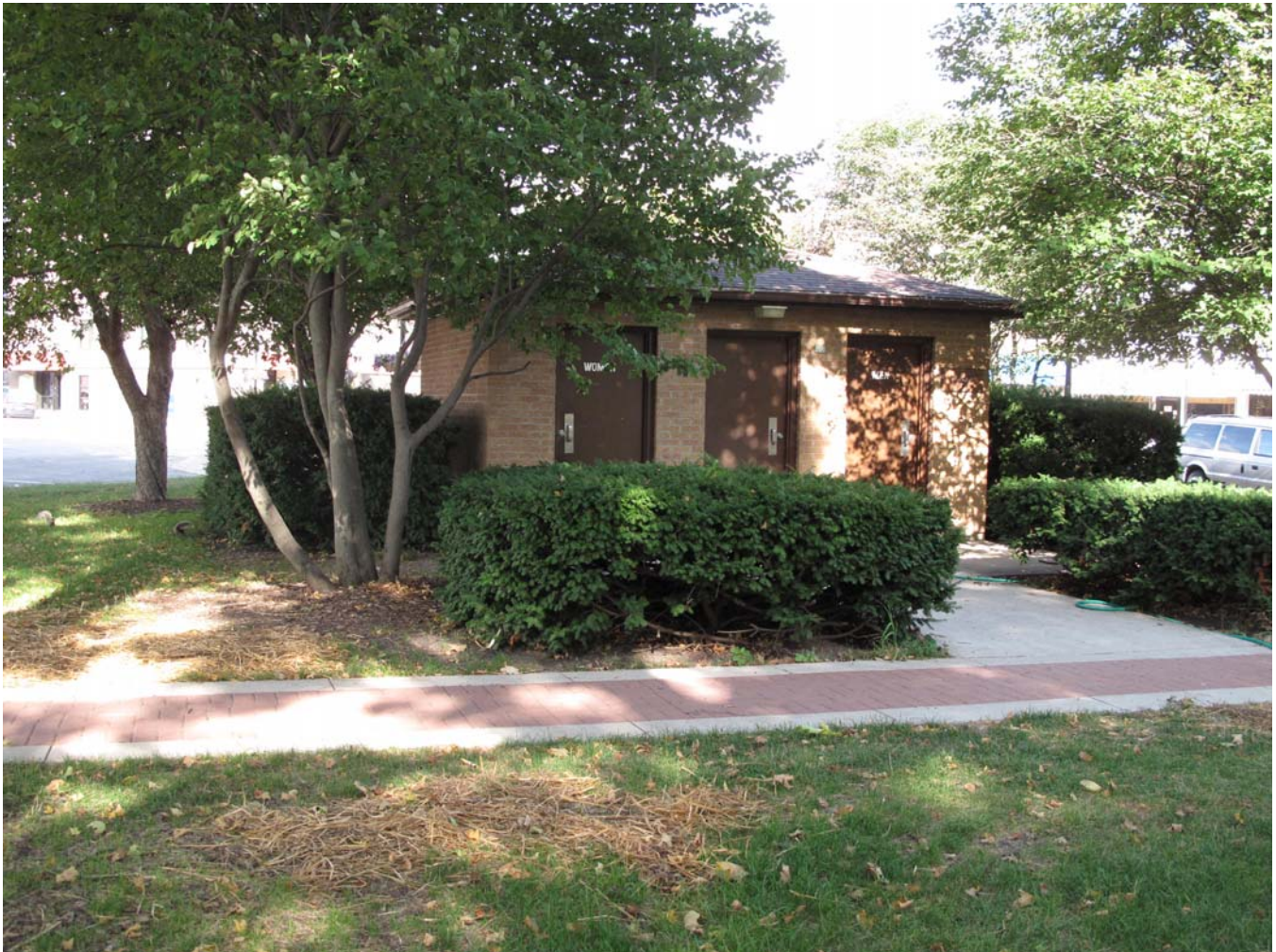
Photograph 92-00493-006 - Rest room building in Central Park, looking northeast (McCarley, September 20, 2011)
