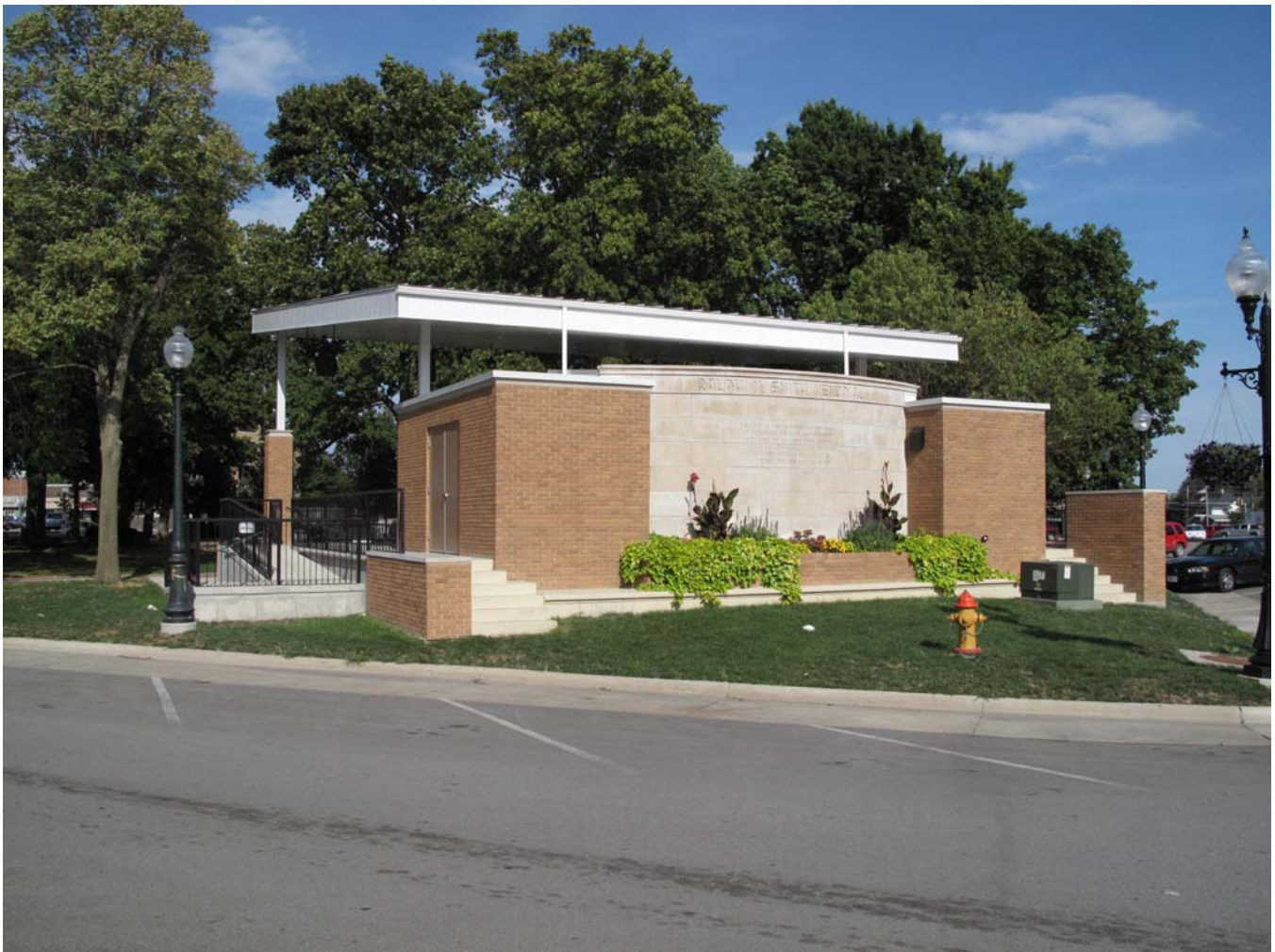
Photograph 92-00493-005 - Historic lamp post and rebuilt bandstand at southwest corner of Central Park, looking northeast (McCarley, September 20, 2011)
