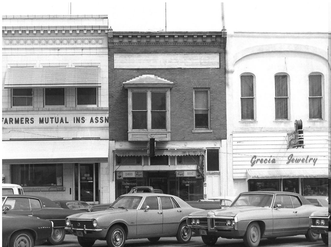
Building in 1971 (Wagner 1971)
