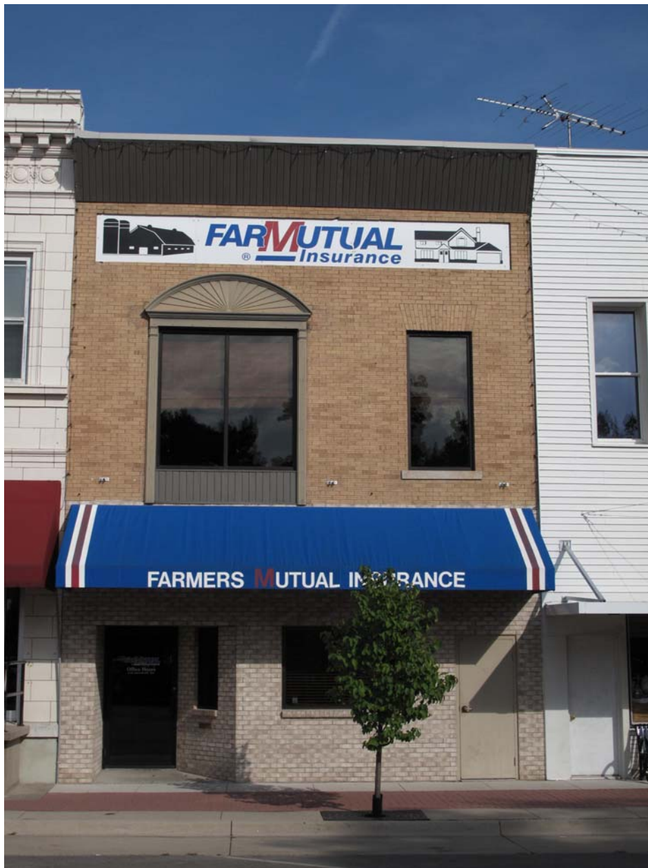
Photograph 92-00509-001 - West elevation, looking east (McCarley, September 20, 2011)
