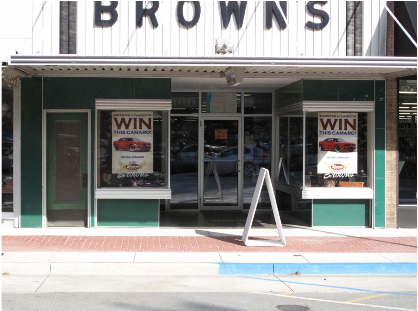
Photograph 92-00512-002 - Detail of storefront, looking east (McCarley, September 20, 2011)
