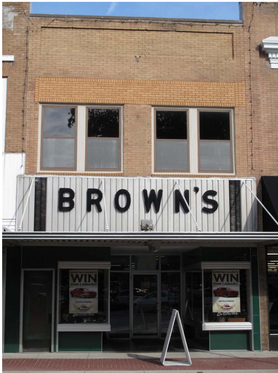
Photograph 92-00512-001 - West elevation, looking east (McCarley, September 20, 2011)
