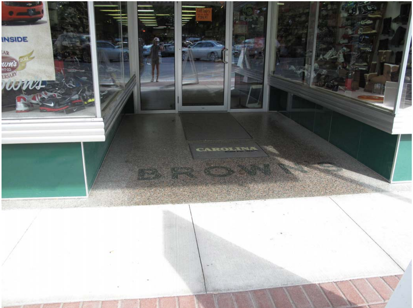
Photograph 92-00512-003 - Detail of storefront floor, looking east (McCarley, September 20, 2011)
