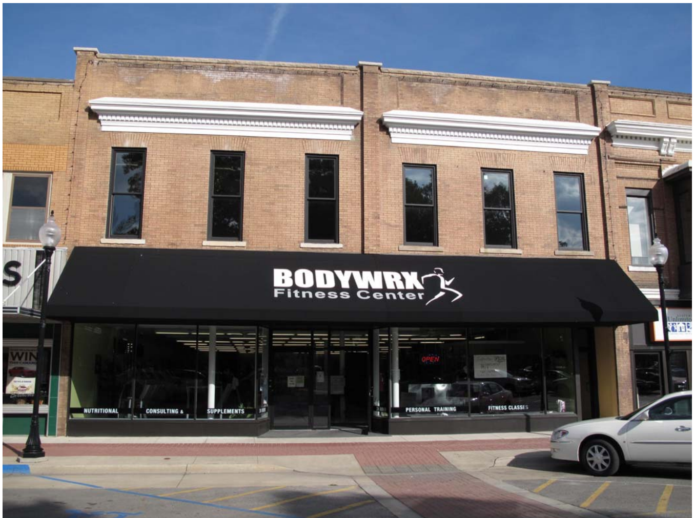
Photograph 92-00513-001 - West elevation, looking east (McCarley, September 20, 2011)
