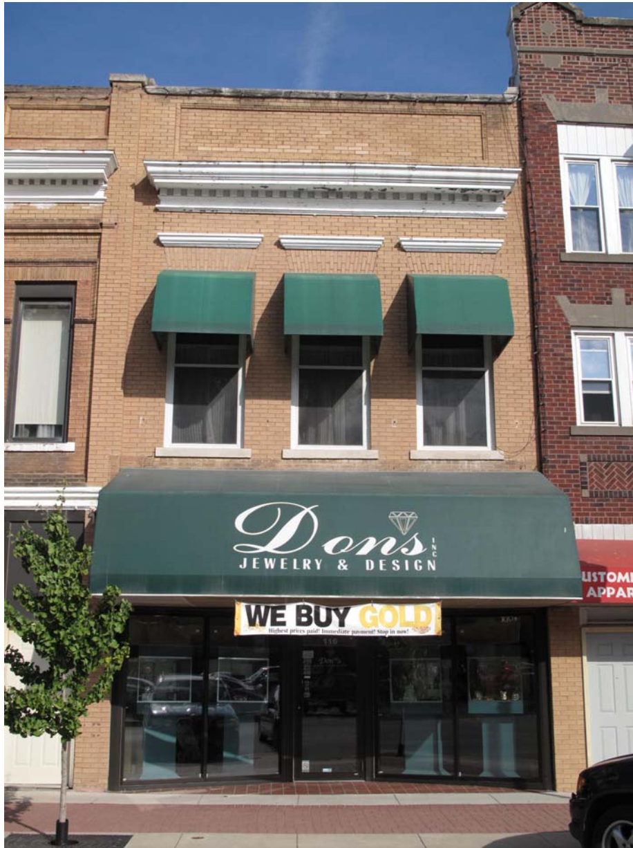
Photograph 92-00515-001 - West elevation, looking east (McCarley, September 20, 2012)
