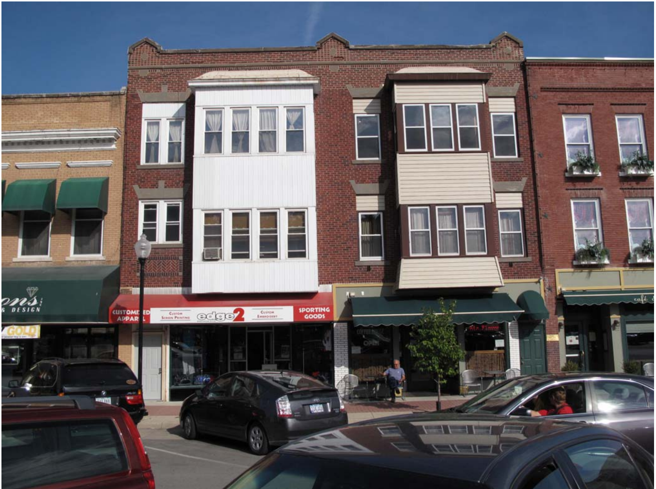
West side (facade) of building, looking east (McCarley, September 20, 2011).
