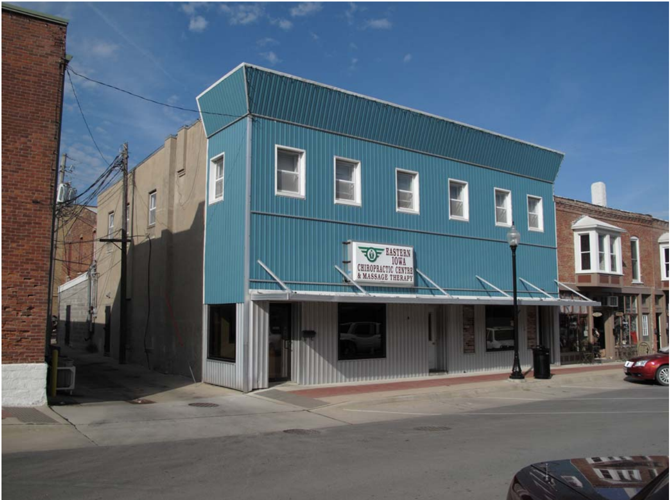
Photograph 92-00595-001 - West and south elevations, looking northeast (McCarley, September 20, 2011)
