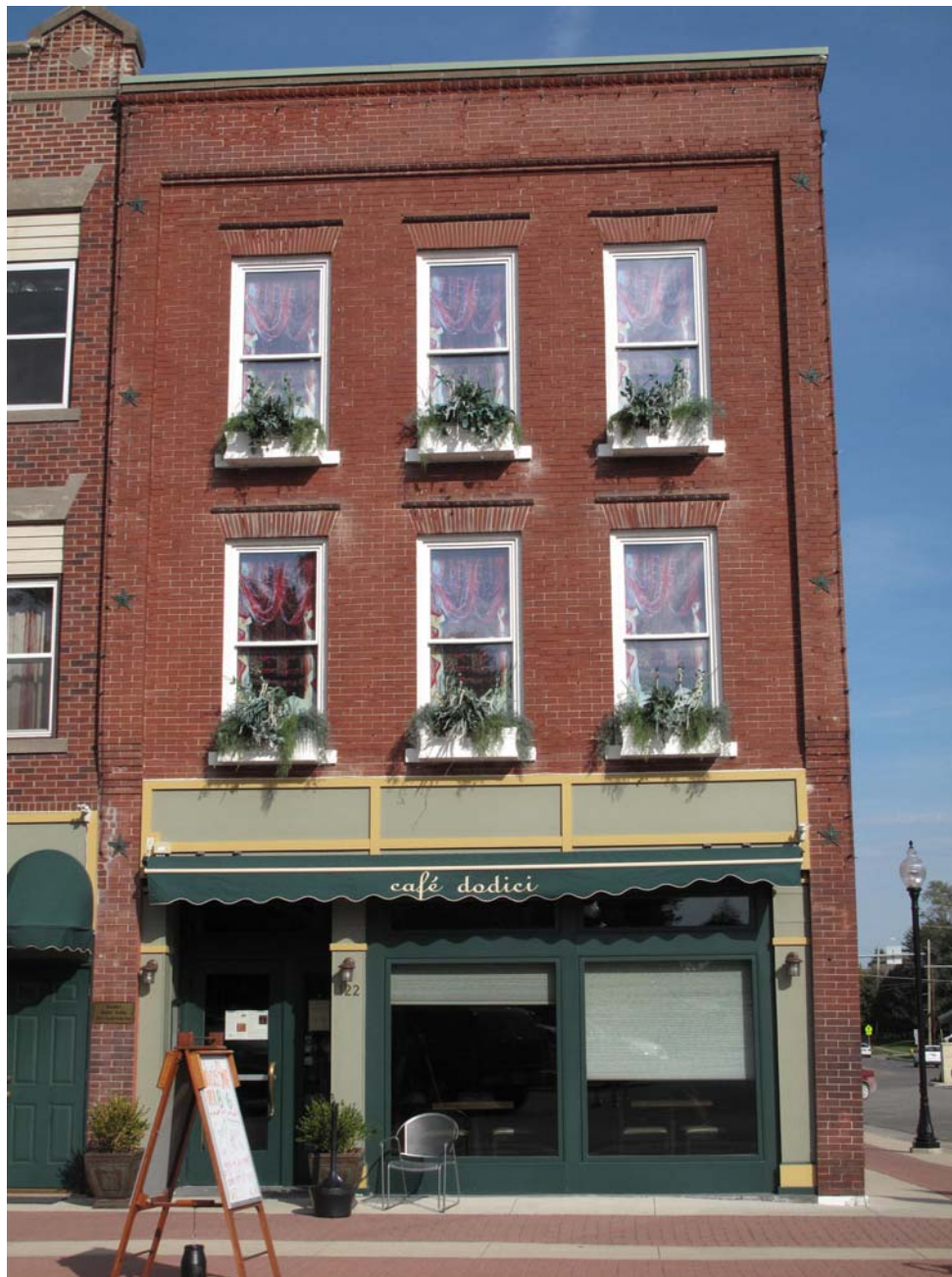
Photograph 92-00517-002 - West elevation, looking east (McCarley, September 20, 2011)
