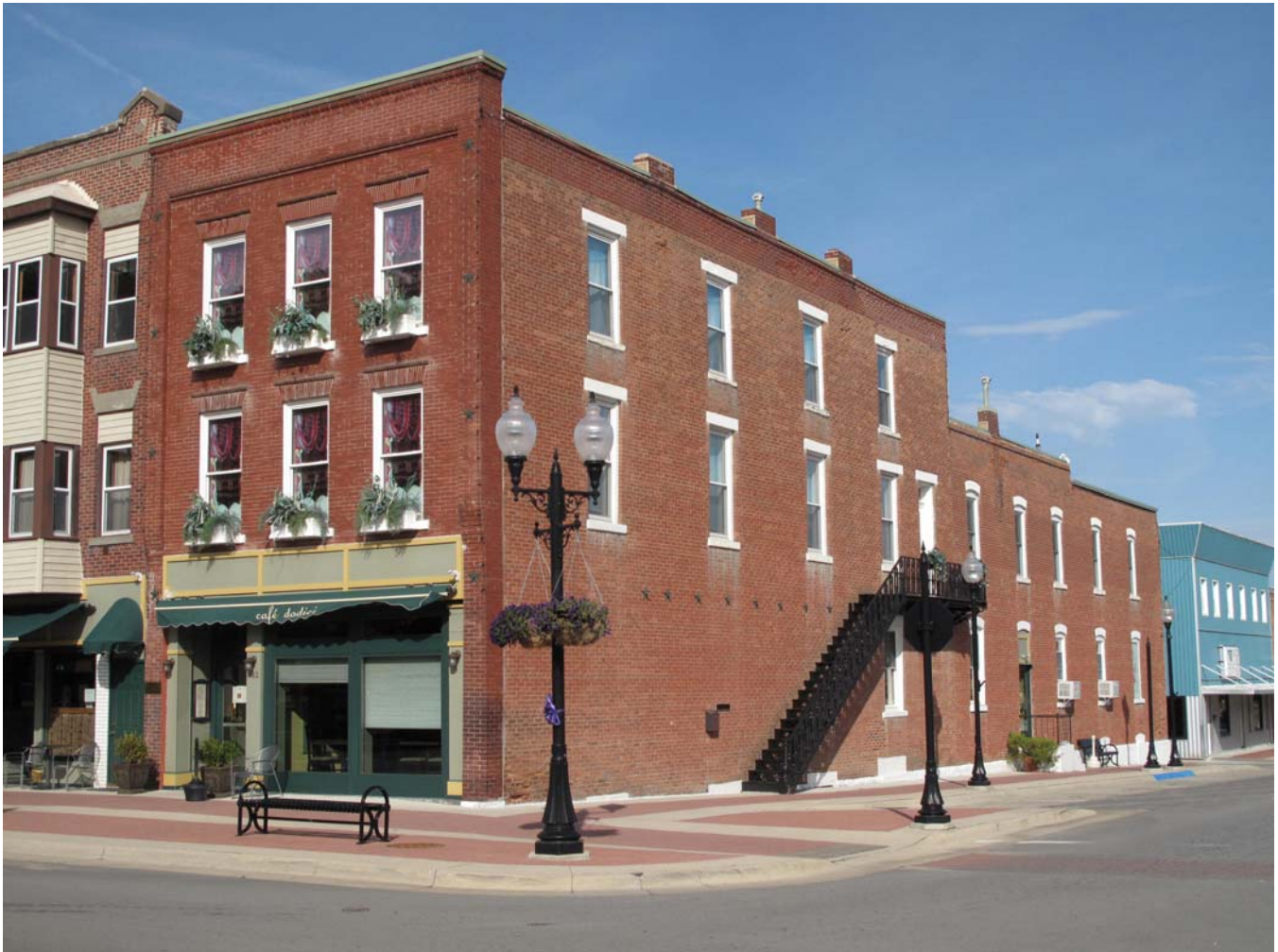
Photograph 92-00517-001 - West and south elevations, looking northeast (McCarley, September 20, 2011)
