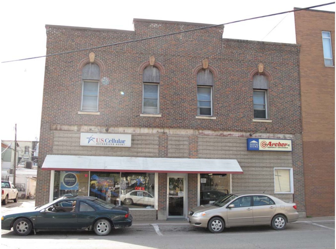
Photograph 92-00494-001 - East elevation, looking west (McCarley, September 20, 2011)
