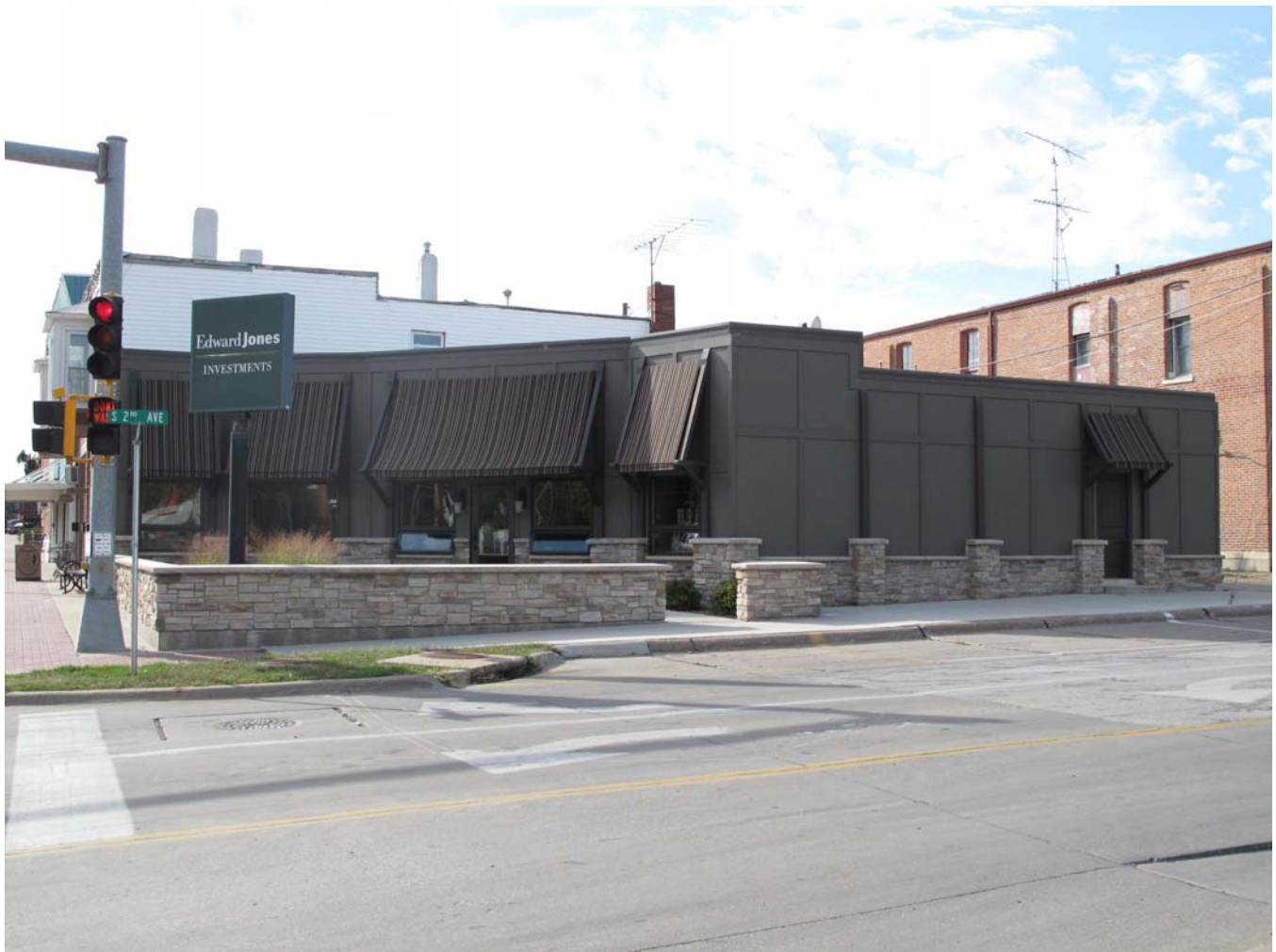
Photograph 92-00599-001 - East elevation of the building, looking west (McCarley, September 20, 2011)
