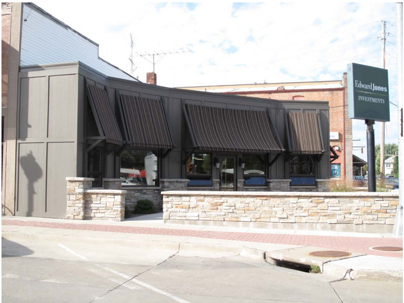
Photograph 92-00599-002 - Southeast elevation of the building, looking north (McCarley, September 20, 2011)
