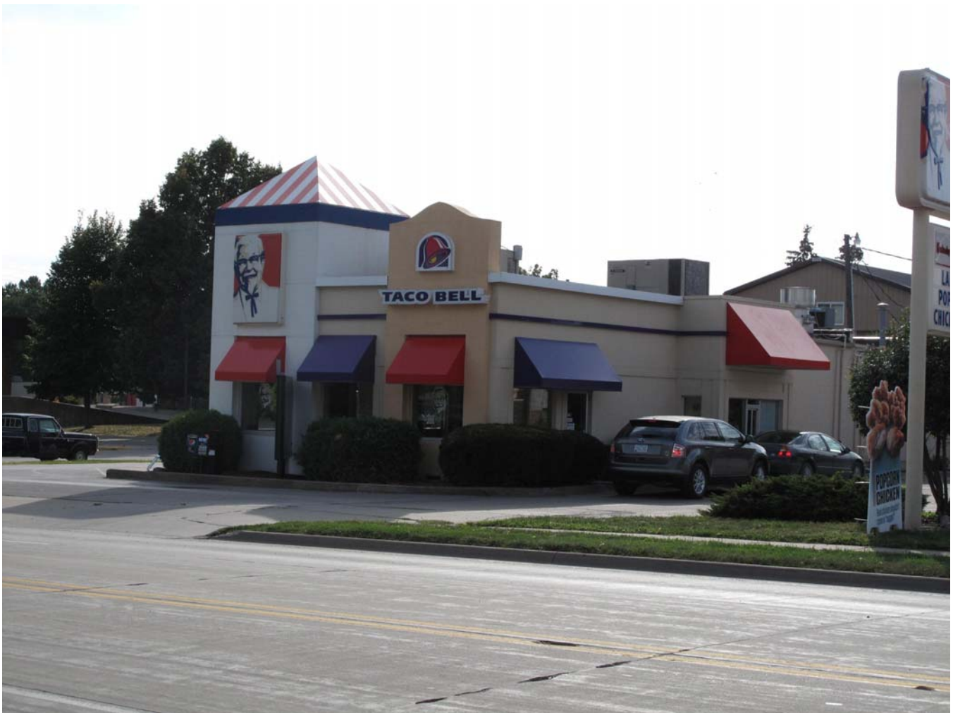
92-00531-001 - East and north elevations, looking southwest (McCarley, September 20, 2011)
