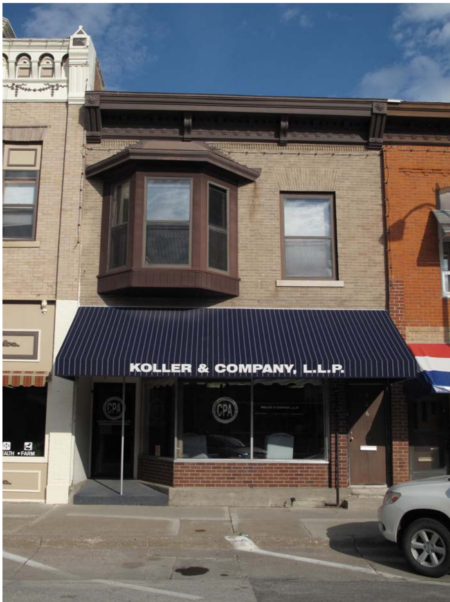
Photograph 92-00519-001 - West elevation, looking east (McCarley, September 20, 2011)
