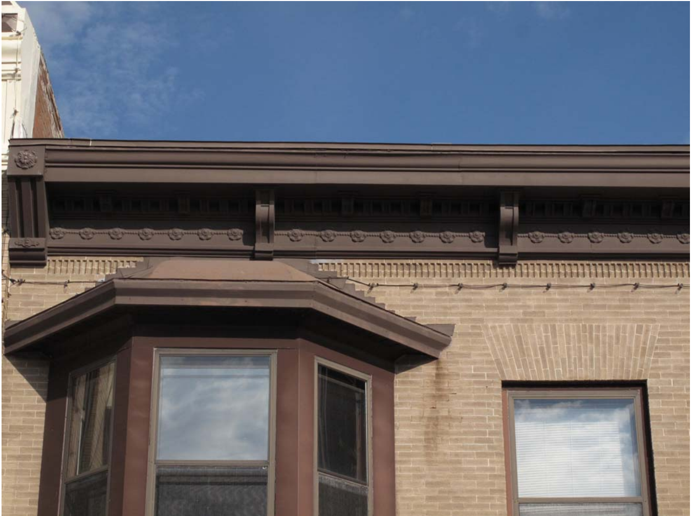
Photograph 92-00519-002 - Detail on west elevation, looking east (McCarley, September 20, 2011)
