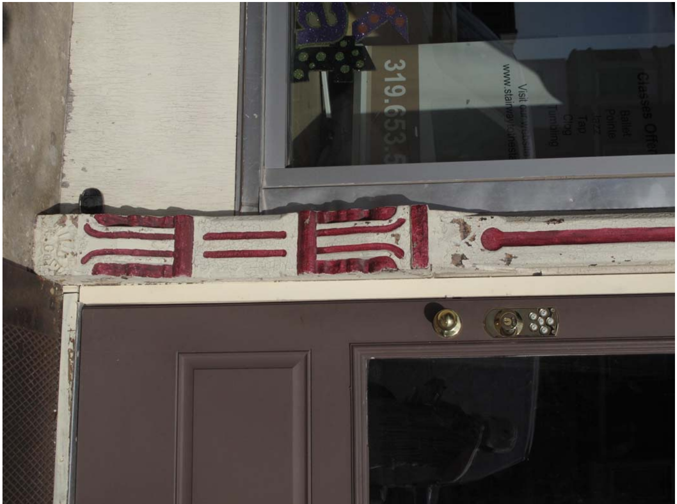
Photograph 92-00518-008 - Middle column of 202 storefront, looking east (McCarley, September 20, 2011)
