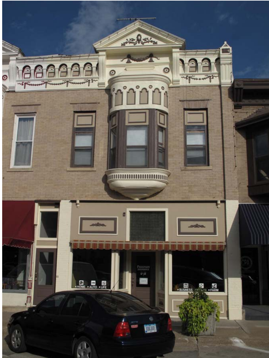
Photograph 92-00518-003 - Detail of 204 section, looking east (McCarley, September 20, 2011)
