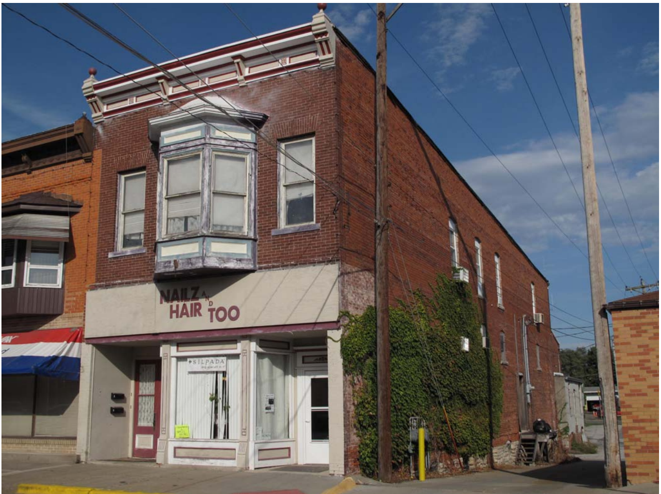
Photograph 92-00521-001 - West and south elevations, looking northeast (McCarley, September 20, 2011)
