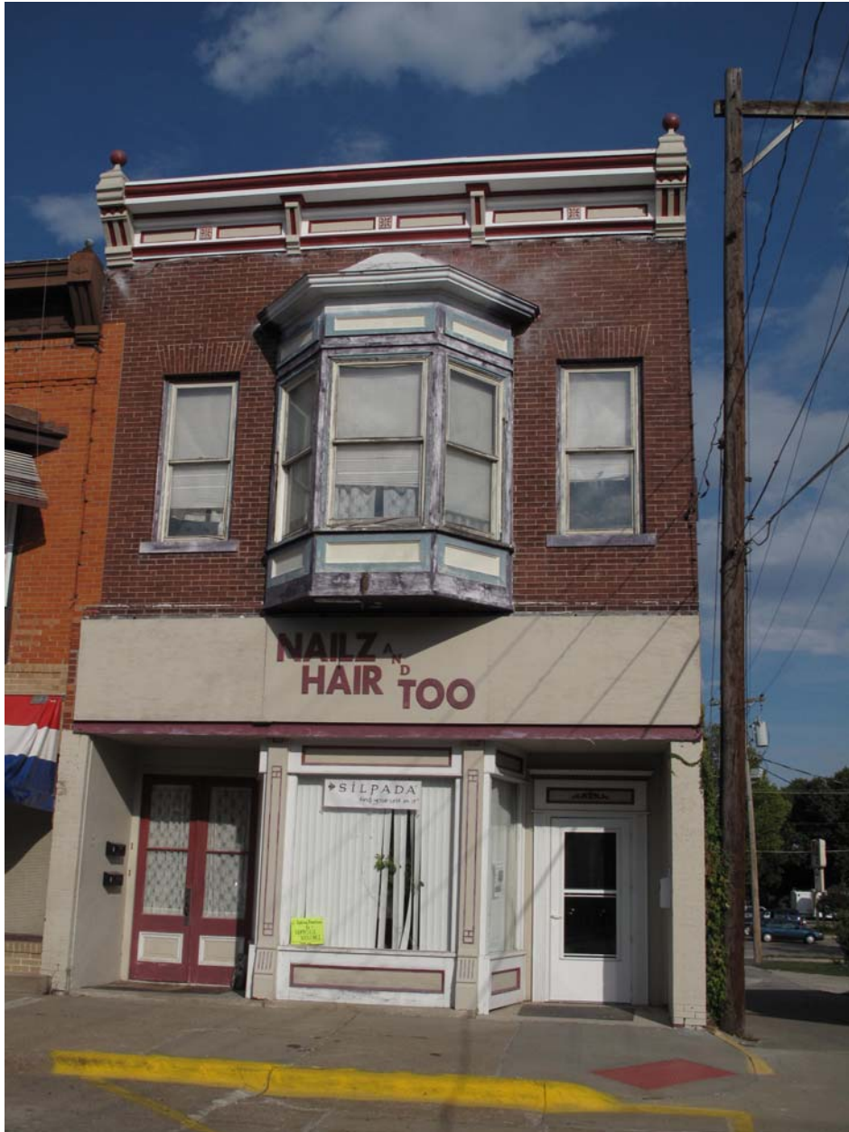
Photograph 92-00521-003 - West elevation, looking east (McCarley, September 20, 2011)
