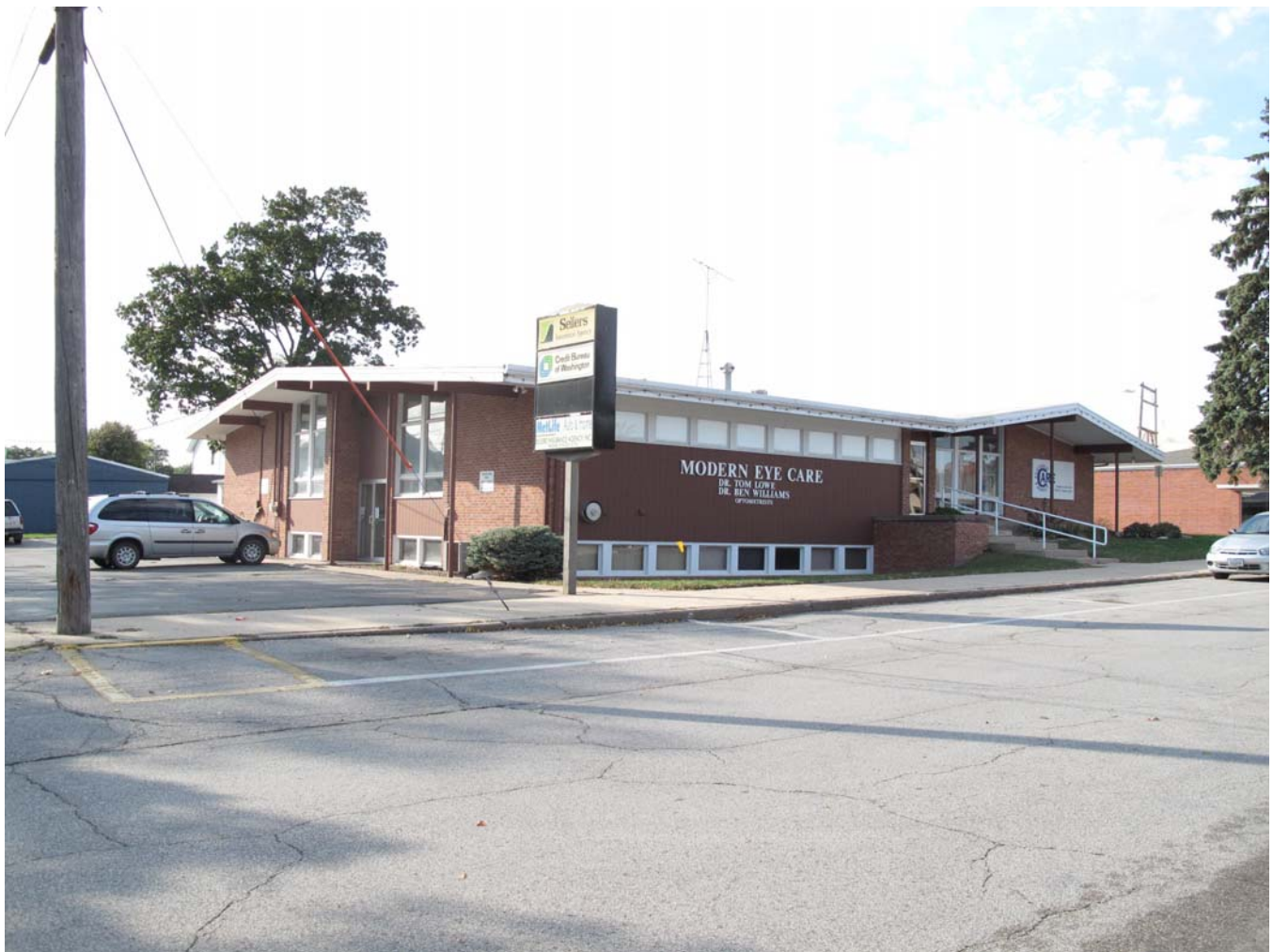
Photograph 92-00529-001 - South and east elevations, looking northwest (McCarley, September 20, 2011)
