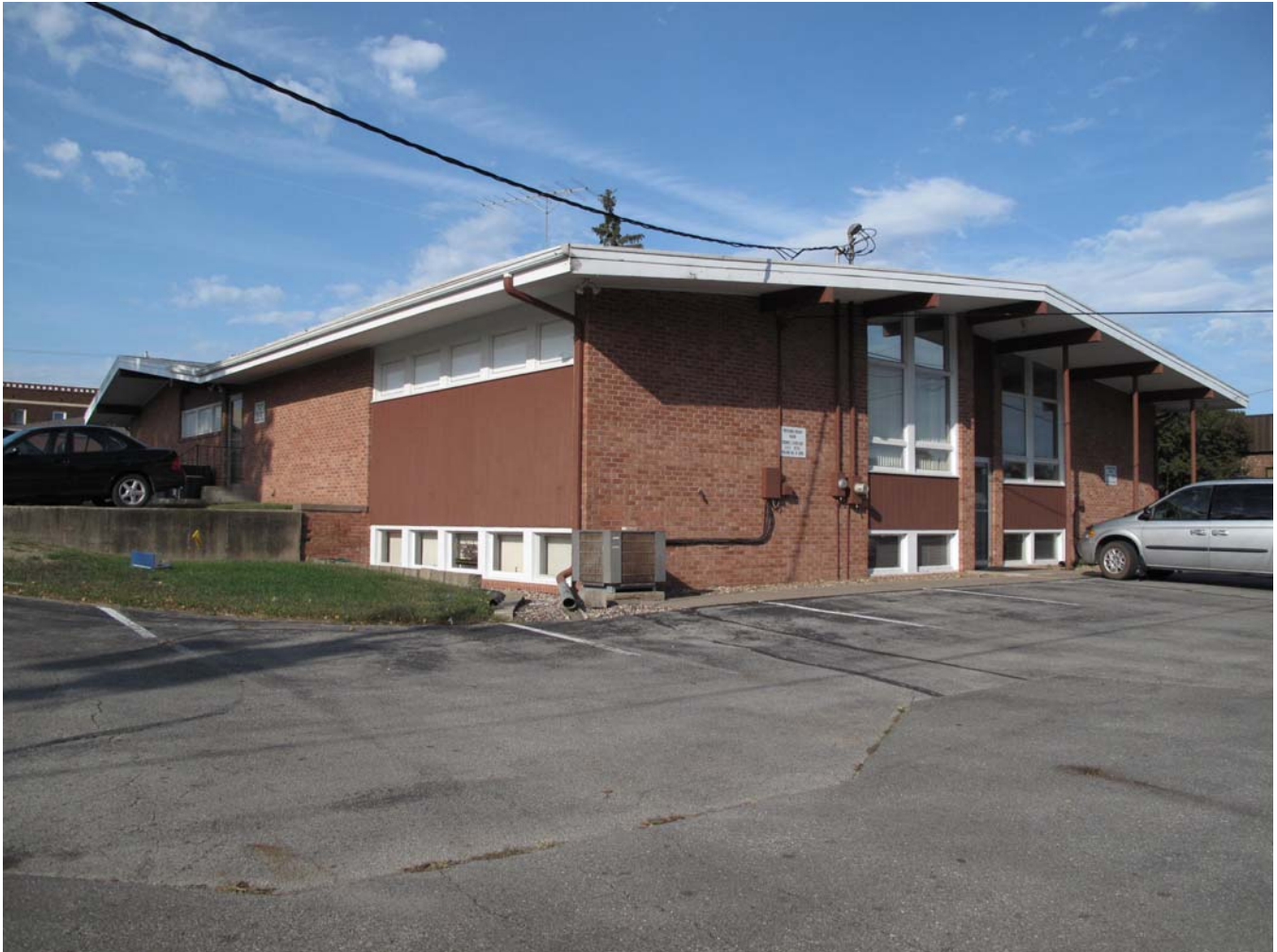
Photograph 92-00529-004 - West and south elevations, looking northeast (McCarley, September 20, 2011)
