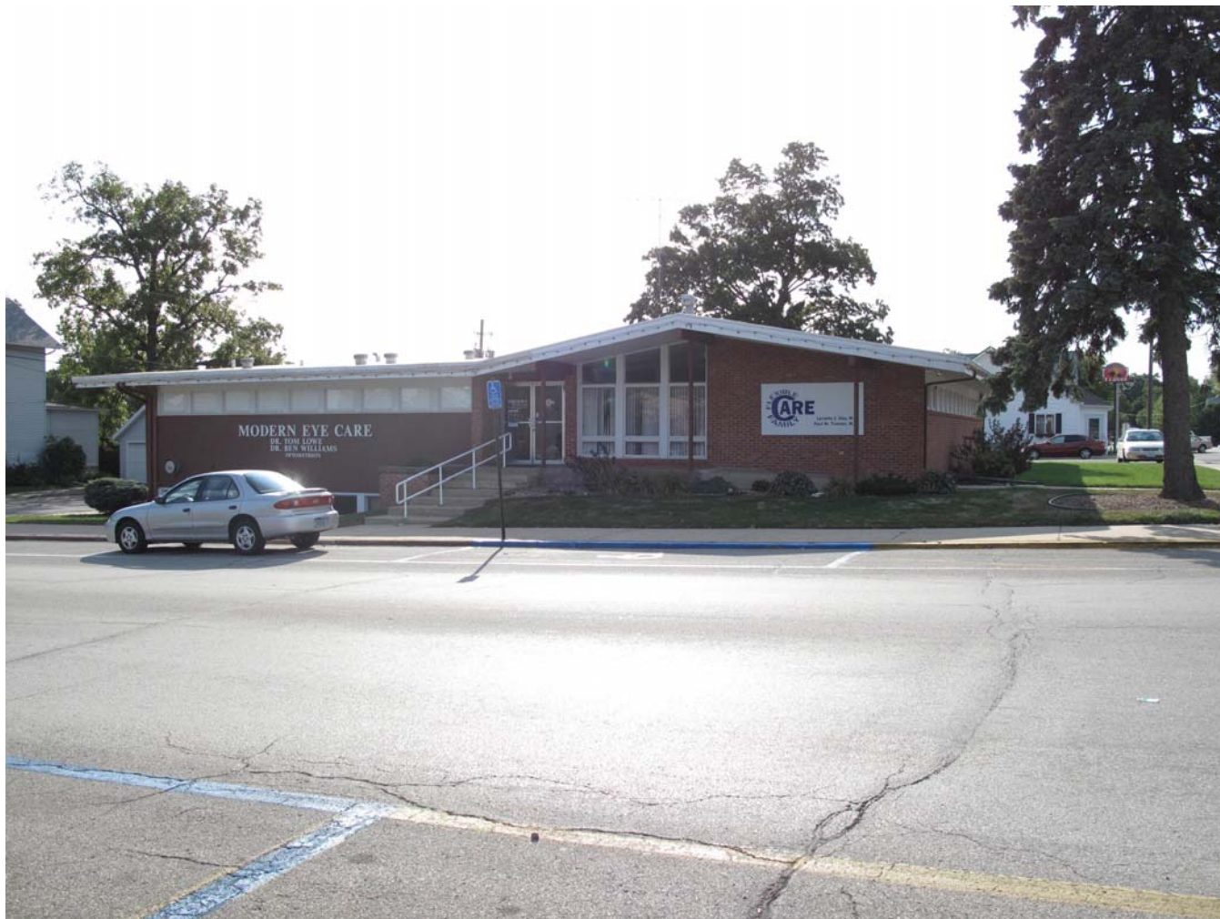
Photograph 92-00529-002 - East elevation, looking west (McCarley, September 20, 2011)
