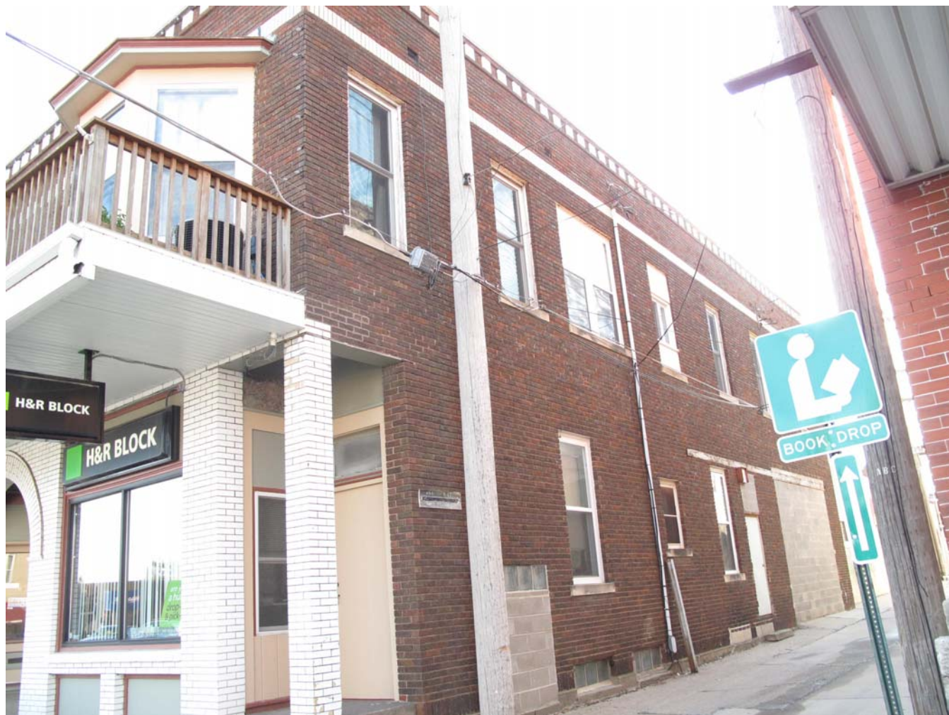
92-00523-004 - North elevation, looking southwest (McCarley, September 20, 2011)
