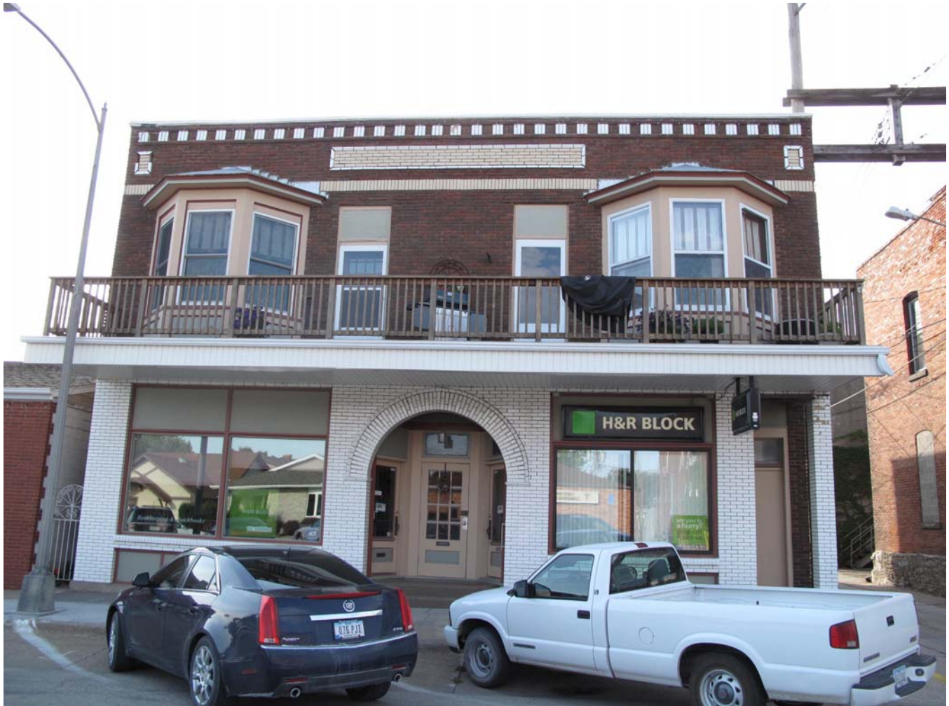
92-00523-002 - East elevation, looking west (McCarley, September 20, 2011)
