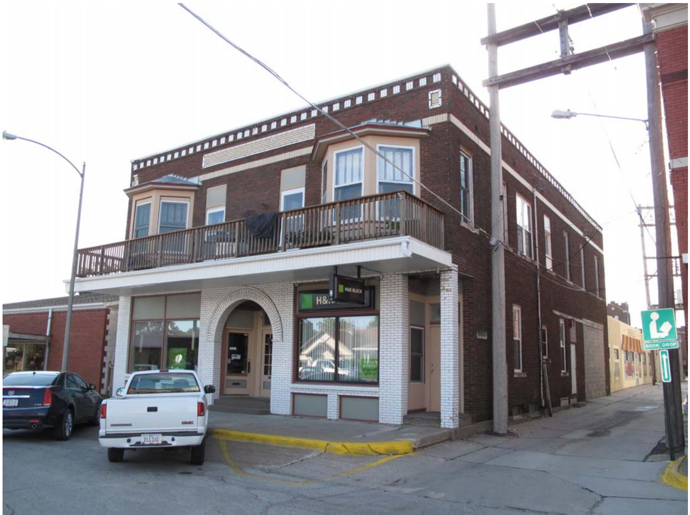
92-00523-001 - East and north elevations, looking southwest (McCarley, September 20, 2011)
