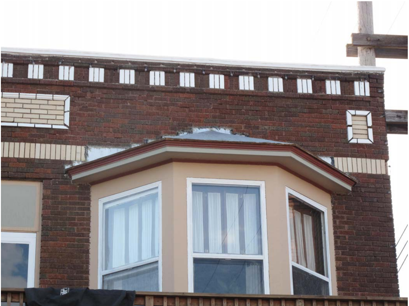
92-00523-003 - Detail on east elevation, looking west (McCarley, September 20, 2011)
