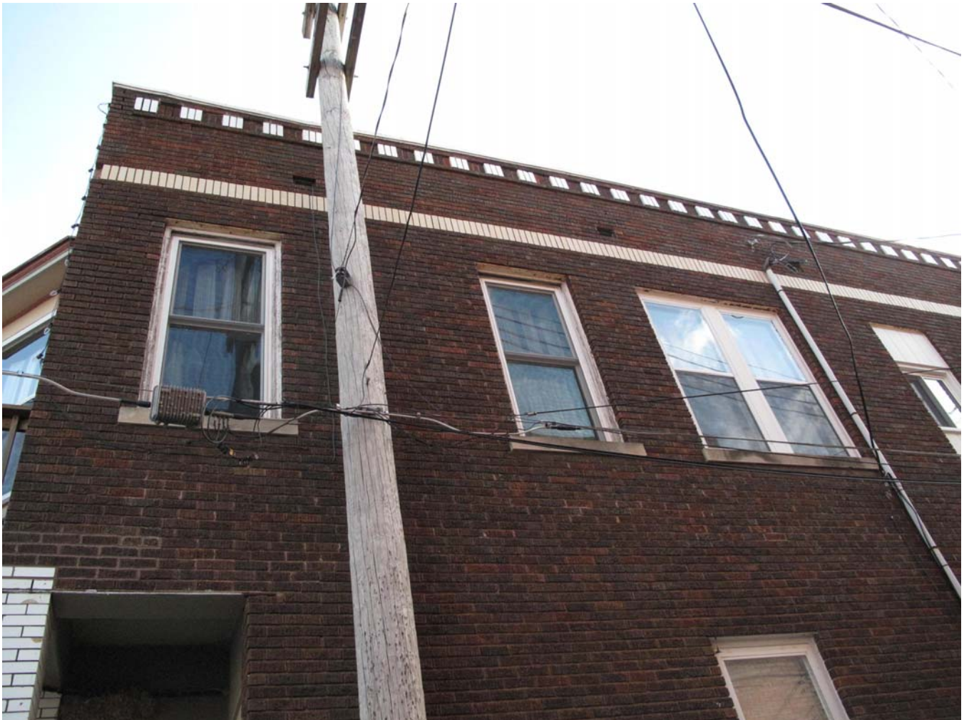
92-00523-005 - Detail on north elevation, looking south (McCarley, September 20, 2011)
