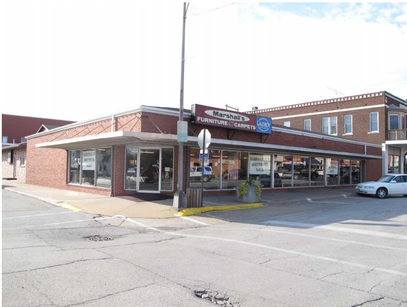
Photograph 92-00525-001 - South and east elevations, looking northwest (McCarley, September 20, 2011)
