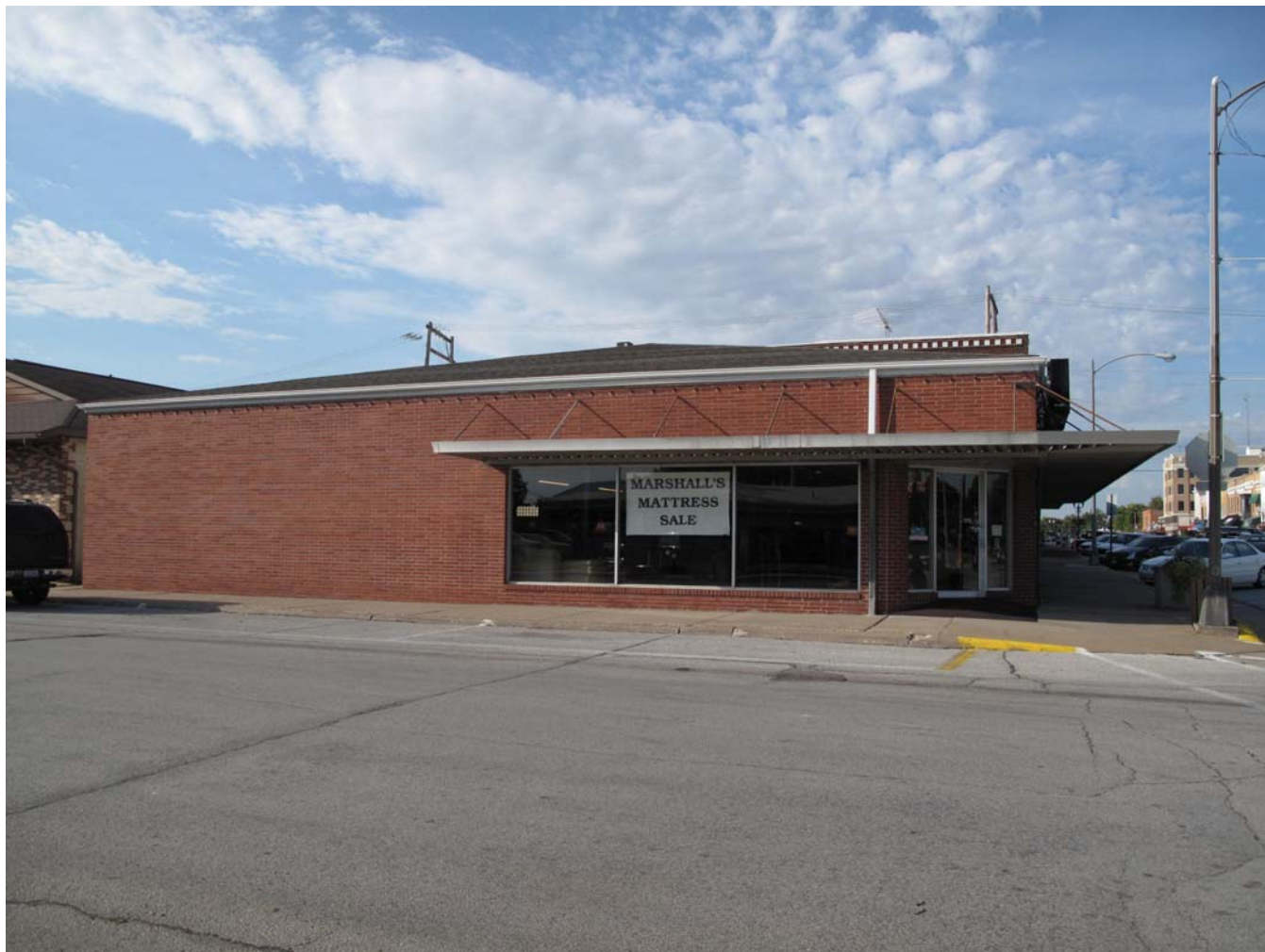
Photograph 92-00525-002 - South elevation, looking north (McCarley, September 20, 2011)
