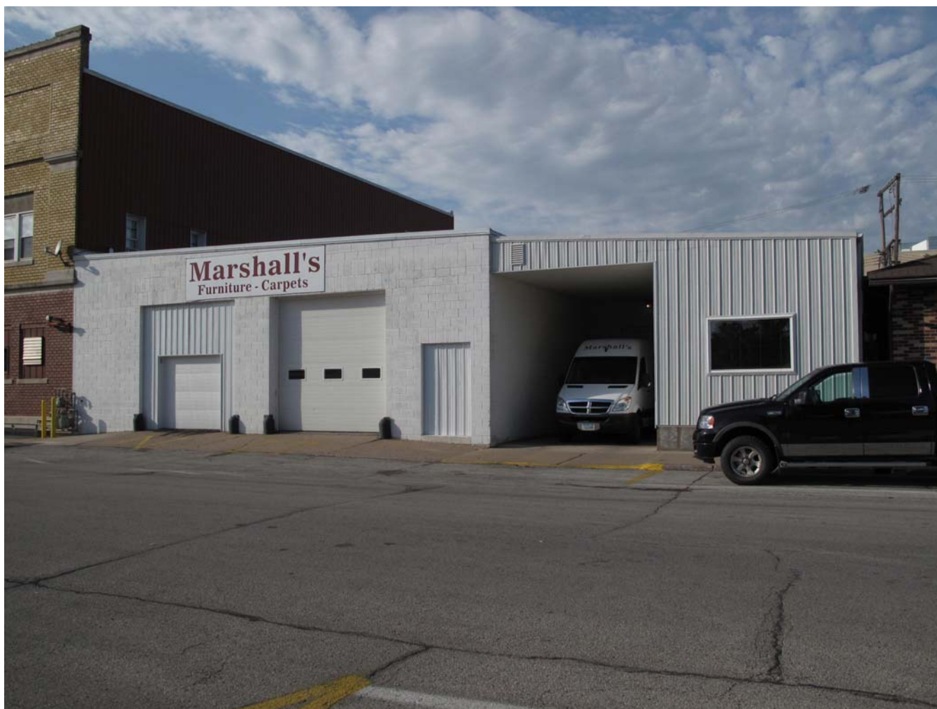
Photograph 92-00527-001 - South elevation, looking north (McCarley, September 20, 2011)
