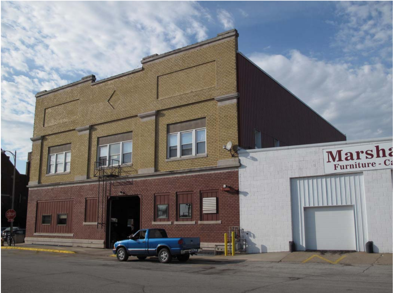
Photograph 92-00574-003 - South and east elevations, looking northwest (McCarley, September 20, 2011)
