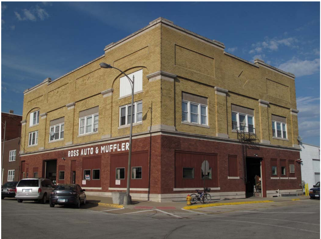
Photograph 92-00574-001 - West and south elevations, looking northeast (McCarley, September 20, 2011)
