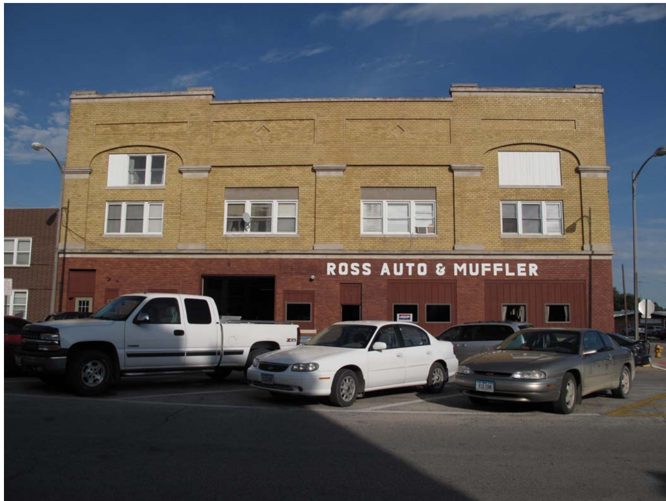
Photograph 92-00574-002 - West elevation, looking east (McCarley, September 20, 2011)
