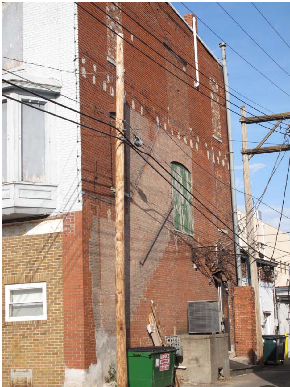
Photograph 92-00596-004 - South elevation, looking northeast (McCarley, September 20, 2011)
