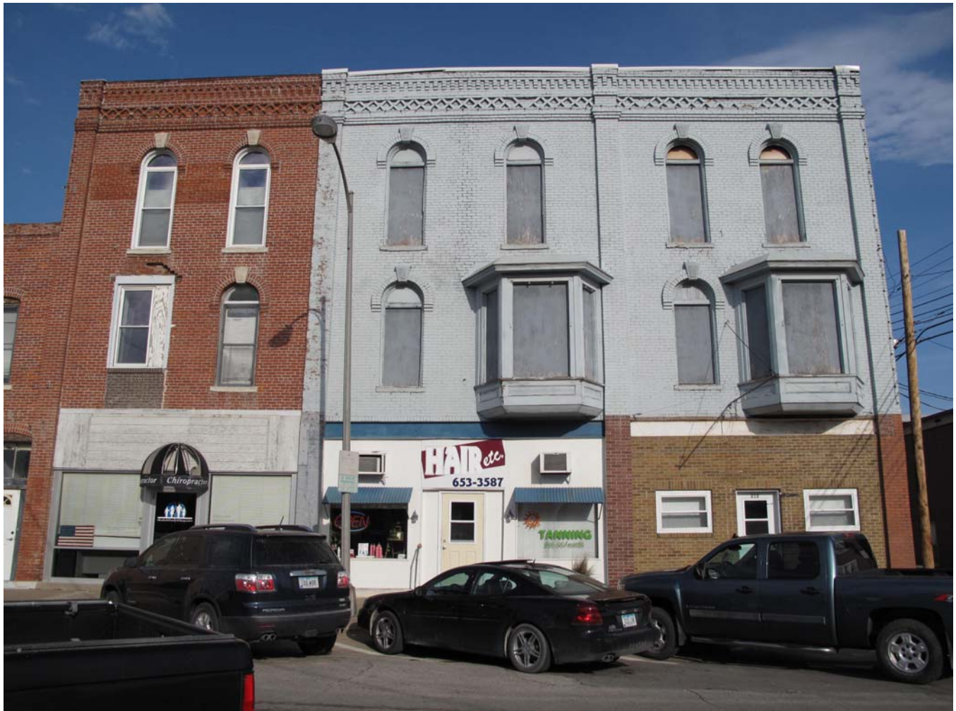
Photograph 92-00596-002 - West elevation, looking east (McCarley, September 20, 2011)
