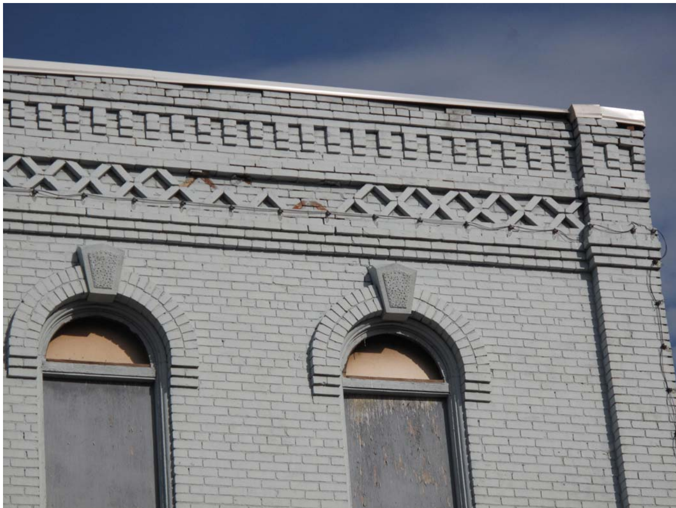
Photograph 92-00596-003 - West elevation, looking east (McCarley, September 20, 2011)
