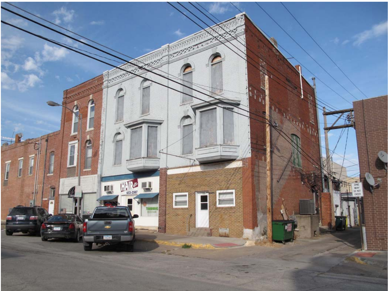
Photograph 92-00596-001 - West and south elevations, looking northeast (McCarley, September 20, 2011)
