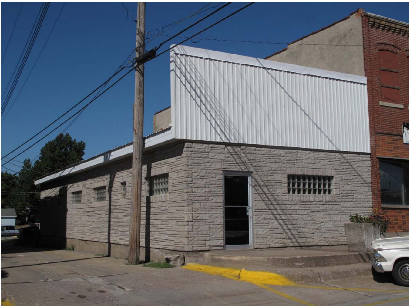
Photograph 92-00571-001 - South and east elevations, looking northwest (McCarley, September 20, 2011)
