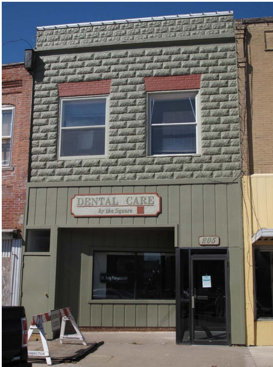
Photograph 92-00567-001 - East facade, looking west (McCarley, September 20, 2011)
