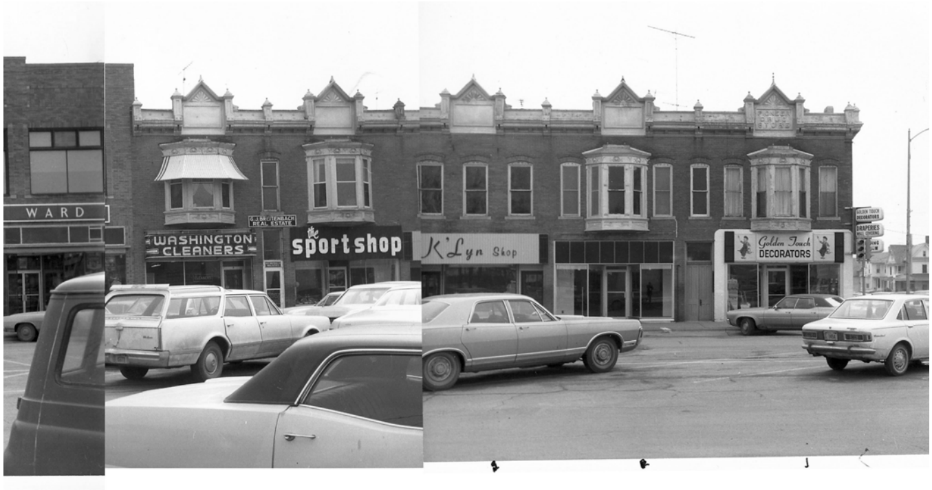
Collage of photos of building in 1971 (Wagner 1971)
