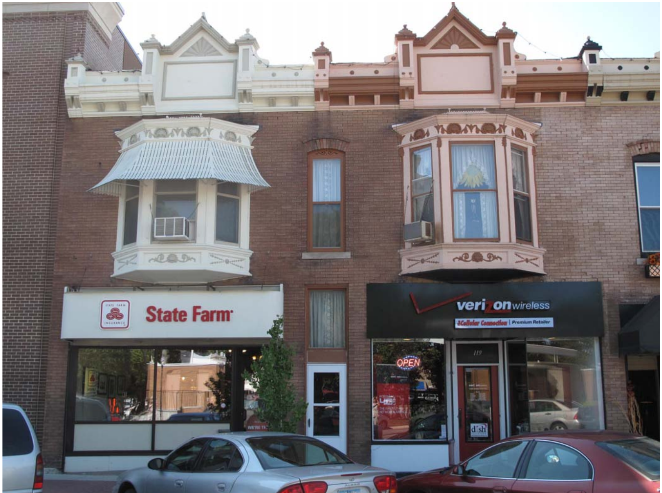
Photograph 92-00605-002 - North elevation of 117-119 W. Washington, looking south (McCarley, September 20, 2011)
