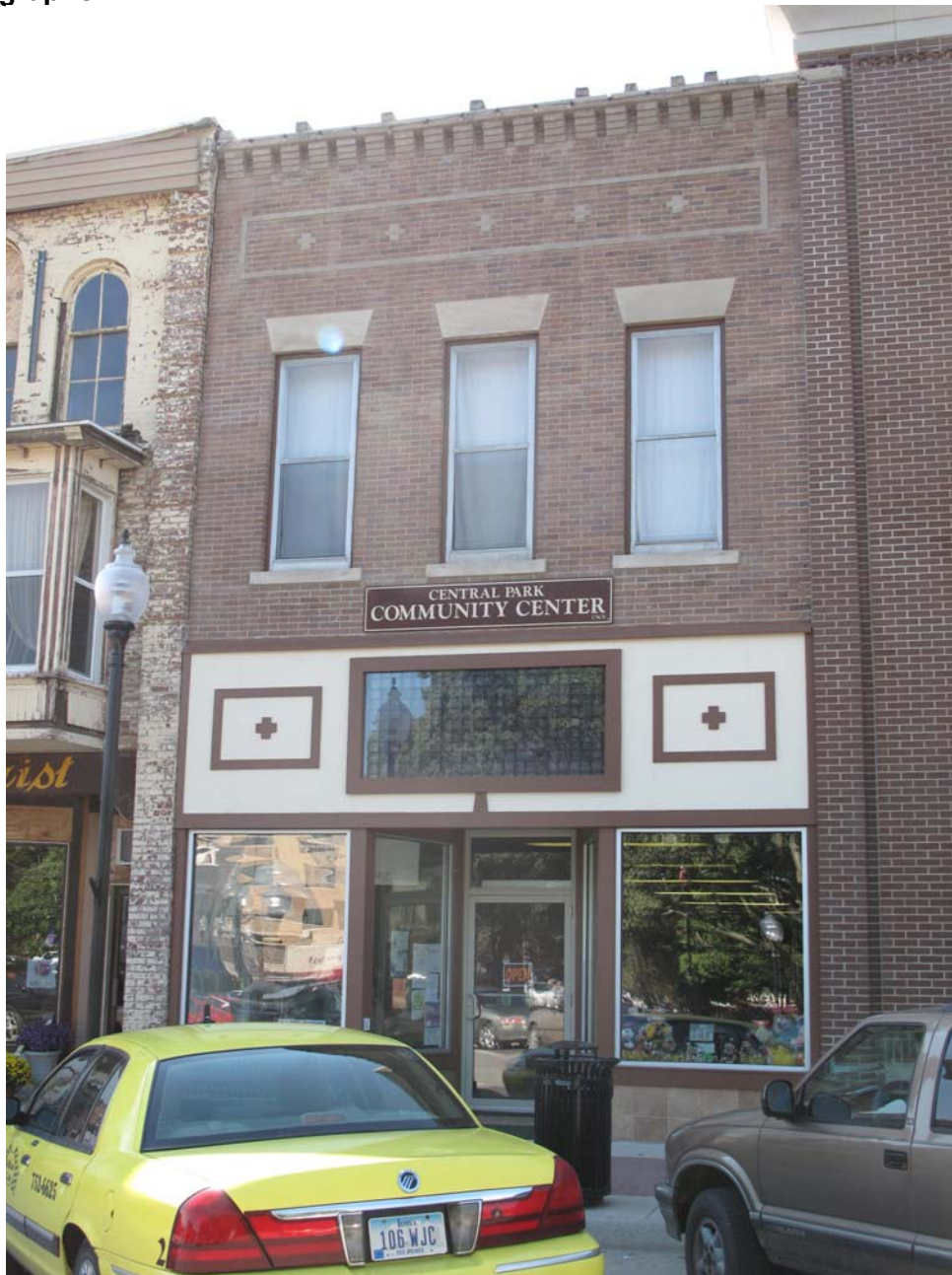
Photograph 92-00603-001 - North elevation, looking south (McCarley, September 20, 2011)
