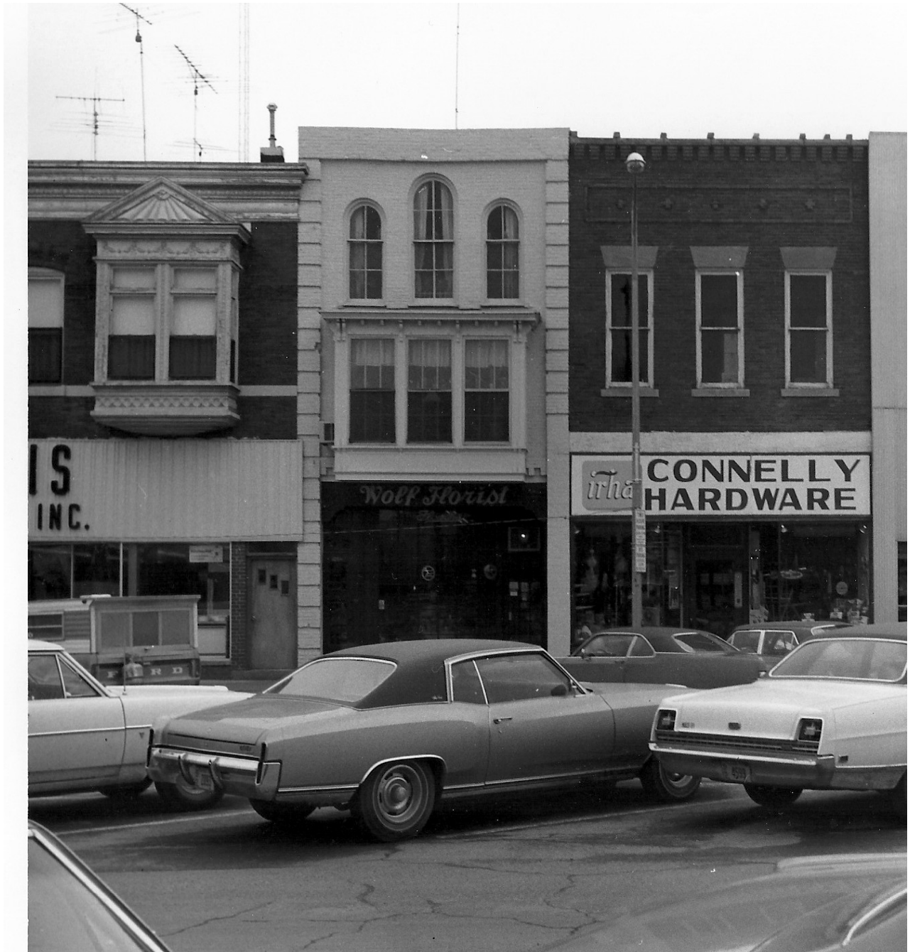
Building in 1971 (Wagner 1971)
