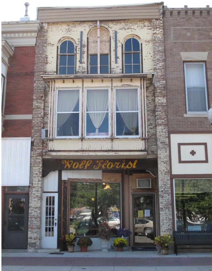
Photograph 92-00602-001 - North elevation, looking south (McCarley, September 20, 2011)
