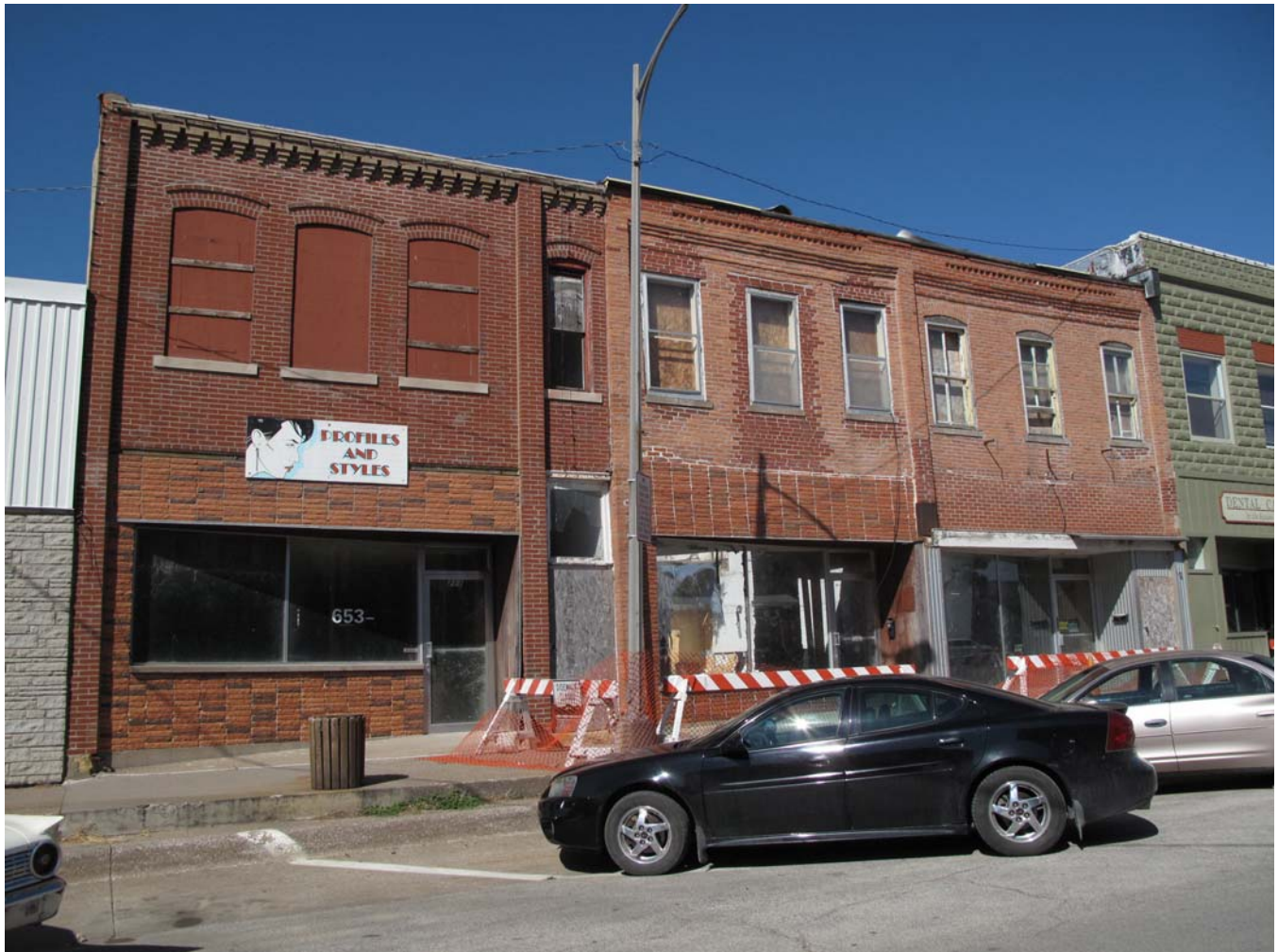
Photograph 92-00570-002 - East elevations of 211-209-207, looking west (September 20, 2011)
