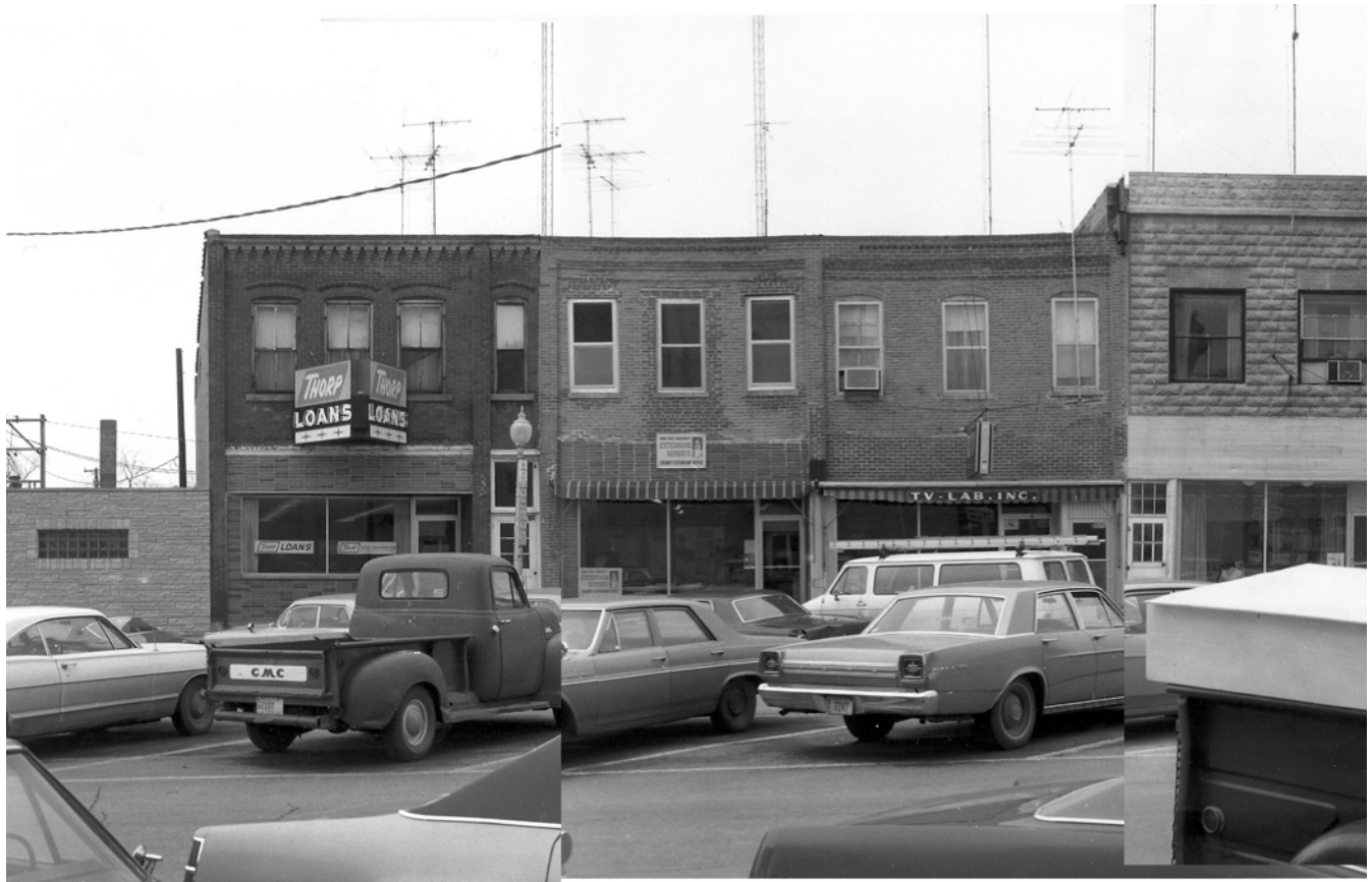
Building in 1971 (Wagner 1971)
