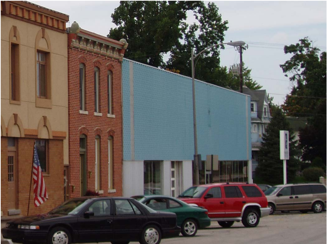
Photograph 92-00614-001 - North elevations of 215-217 and 221-225 W. Washington, looking southwest (McCarley, September 24, 2008)
