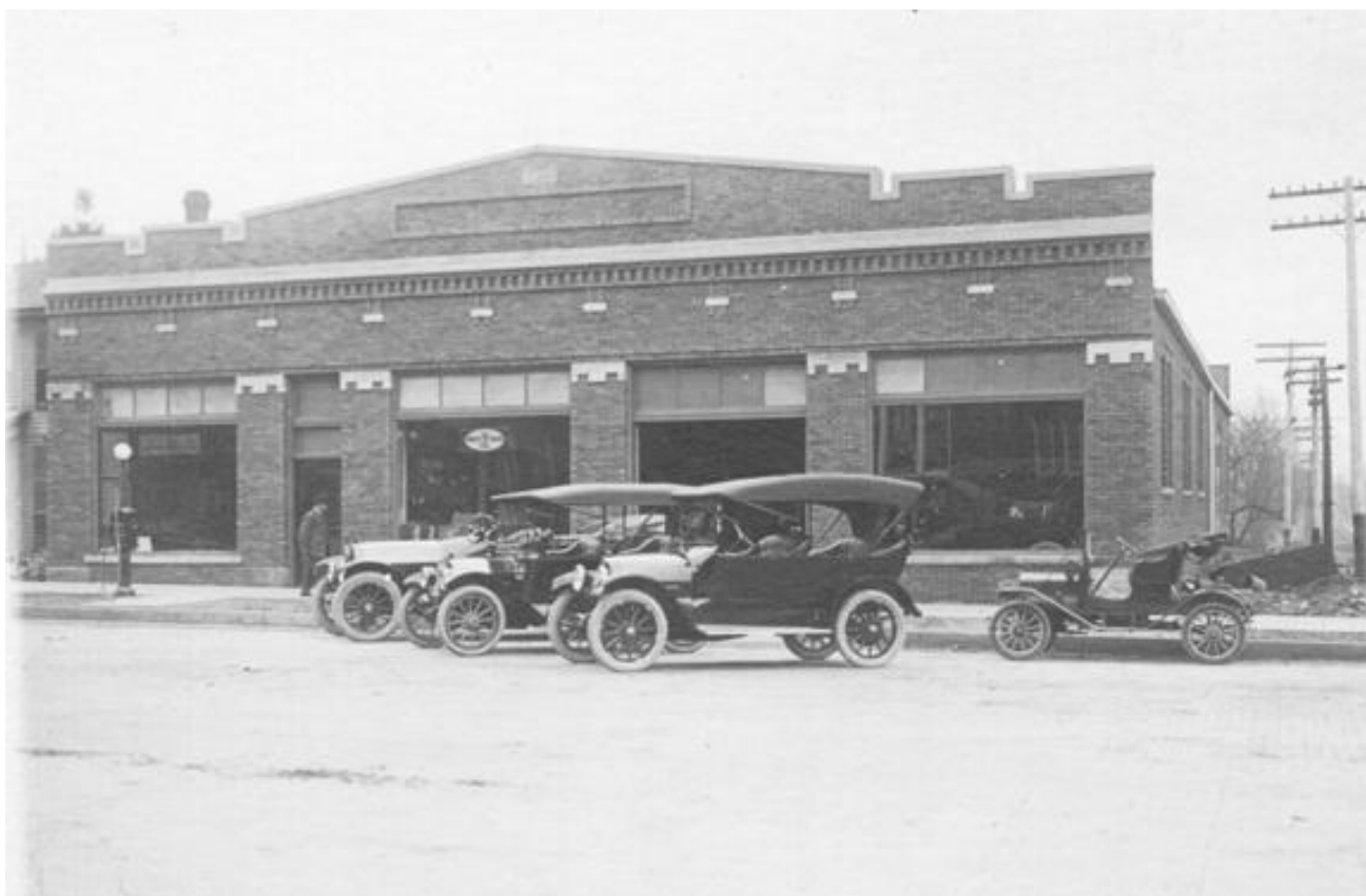
Building in 1920s (from Michael Kramme)
